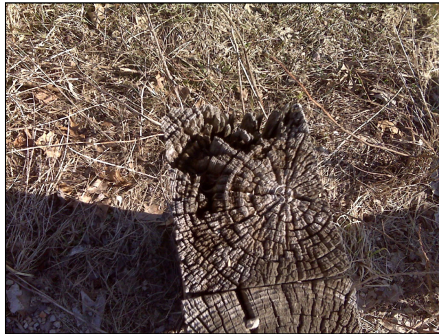
FIGURE 625-8 Rotten Posts
