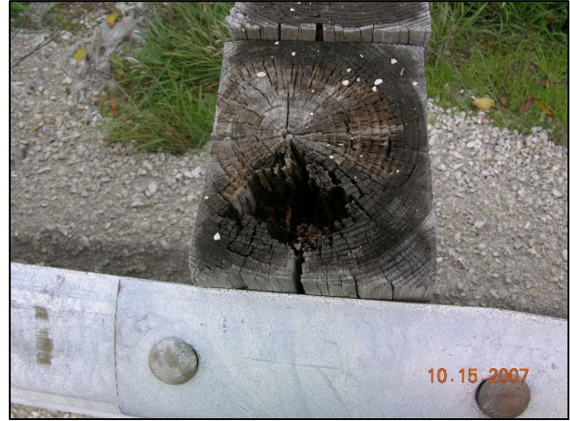
FIGURE 625-7 Rotten Block
