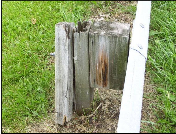
FIGURE 625-6 Damaged Post
