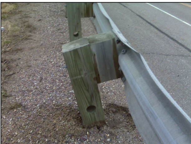
FIGURE 625-5 Post out of Plumb
