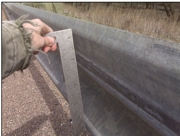
FIGURE 625-9 Rail Damage Examples Flattened Rail
