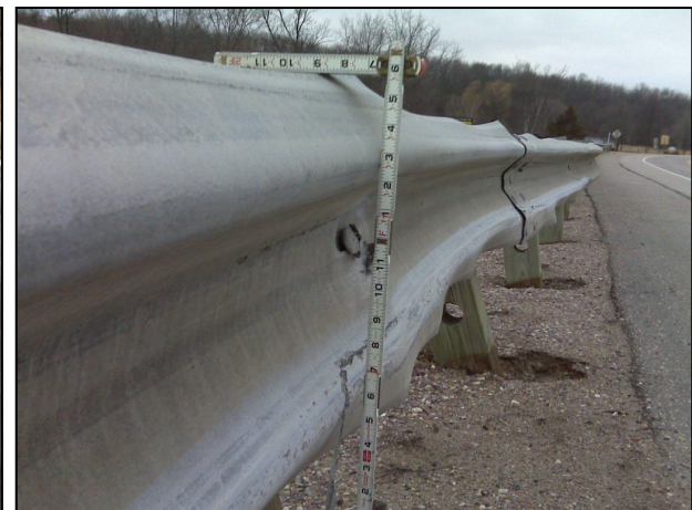
FIGURE 625-9 Rail Damage Examples Flattened Rail
