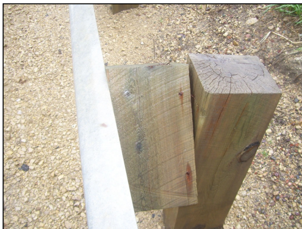
FIGURE 625-4 Twisted Block
