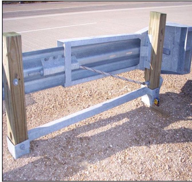
FIGURE 626-4 Ground Strut and Bearing Plate Problems
