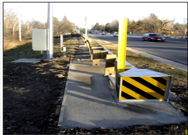
FIGURE 626-15 ITS Pole Can Still be Hit
