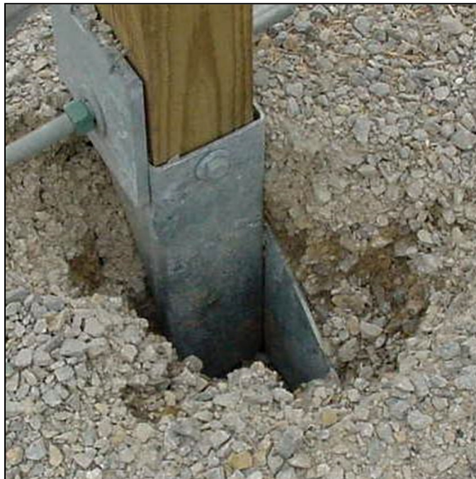
FIGURE 626-3 Poor Compaction/Visible Gaps
