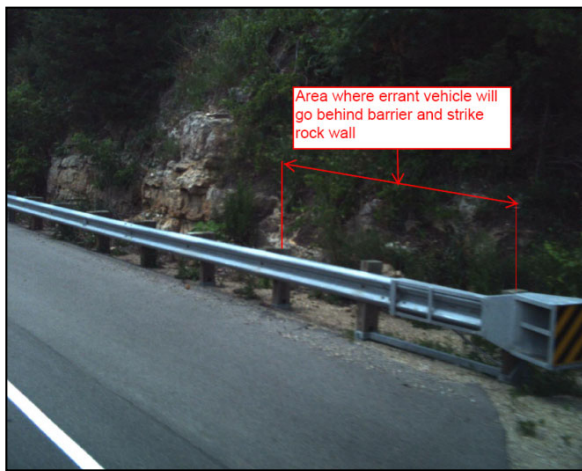
FIGURE 626-14 Rock Wall Can Still be Hit
