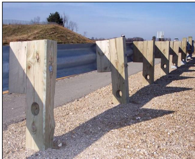
FIGURE 626-1 Breakaway Post
