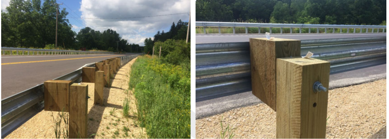
FIGURE 626-16 Block Height Adjustments
