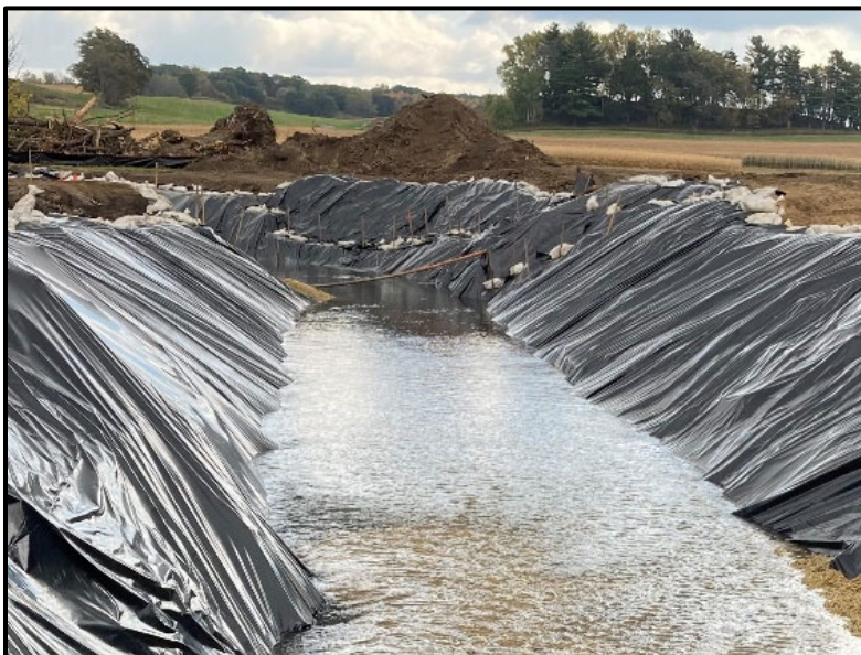
FIGURE 645-1 Polyethylene Sheeting Placement
