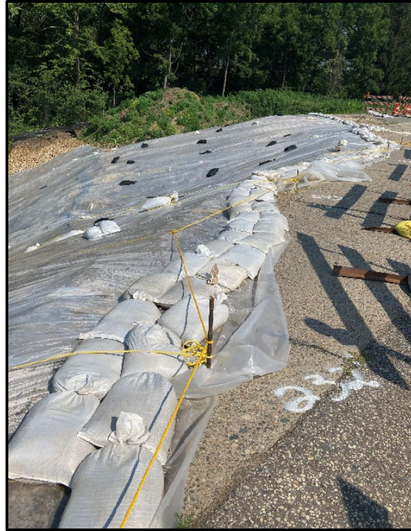
FIGURE 645-2 Securing Polyethylene Sheeting with Sand Bags
