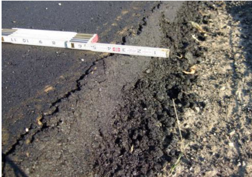
FIGURE 670-4 Cracked Edge
