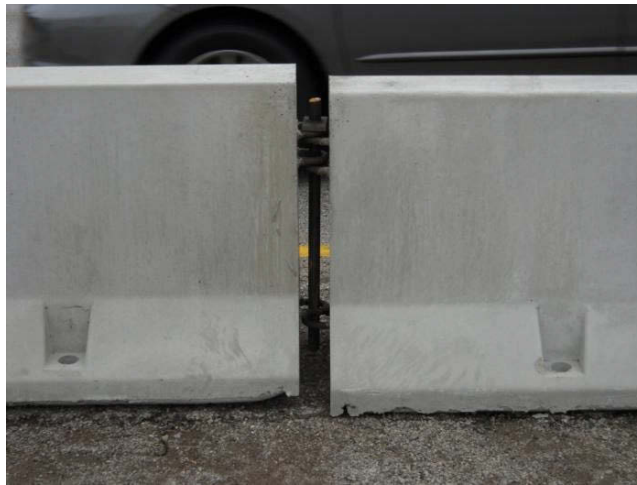
FIGURE 145-22 Improper Connection of 12.5' Temporary Barrier
