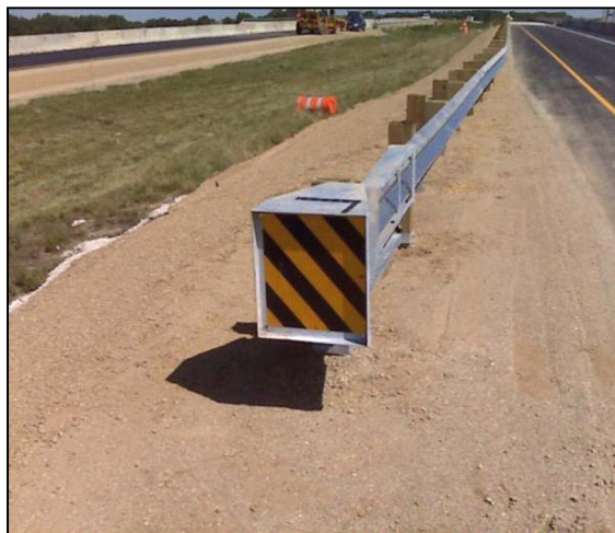
FIGURE 626-6 Desirable Grading
