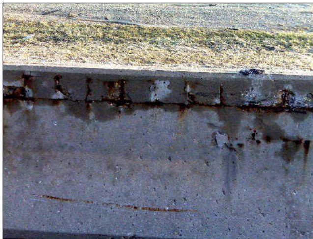
FIGURE 145-10 Exposed Steel Reinforcement
