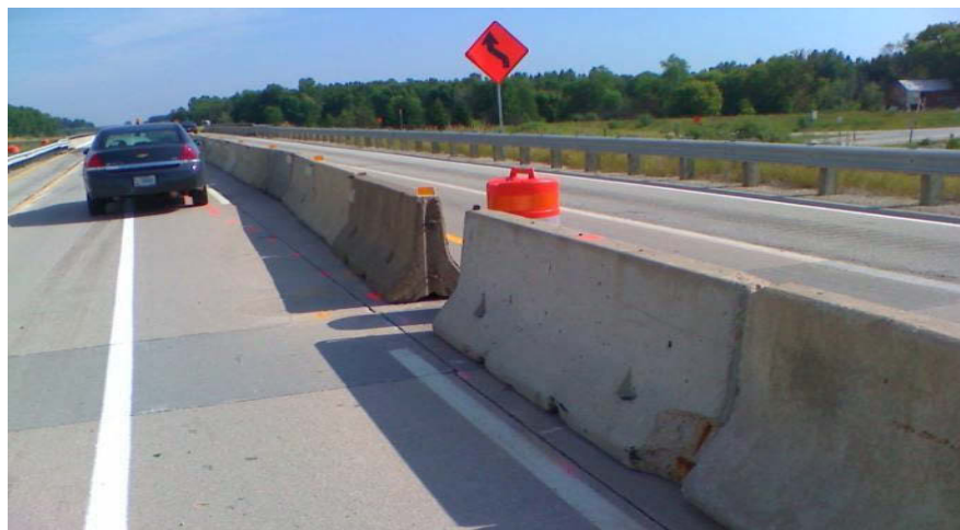
FIGURE 145-20 Gap in Barrier
