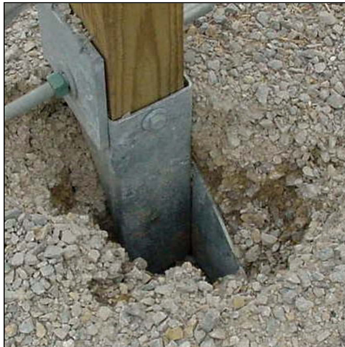
FIGURE 626-3 Poor Compaction/Visible Gaps
