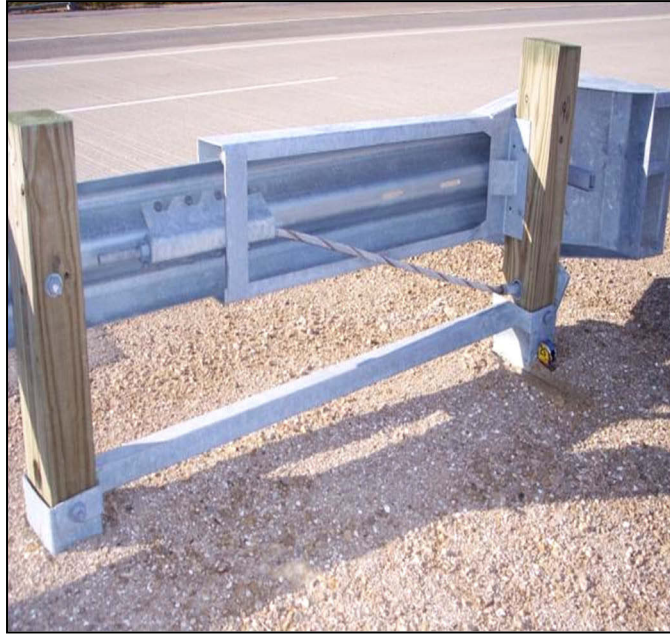
FIGURE 626-4 Ground Strut and Bearing Plate Problems
