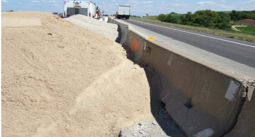
FIGURE 145-21 Insufficient Clearance Behind Temporary Barrier
