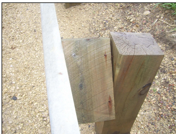
FIGURE 625-4 Twisted Block
