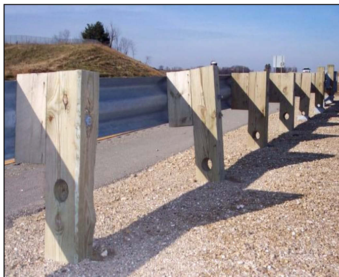
FIGURE 626-1 Breakaway Post
