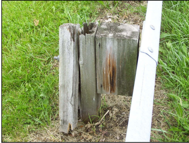
FIGURE 625-6 Damaged Post
