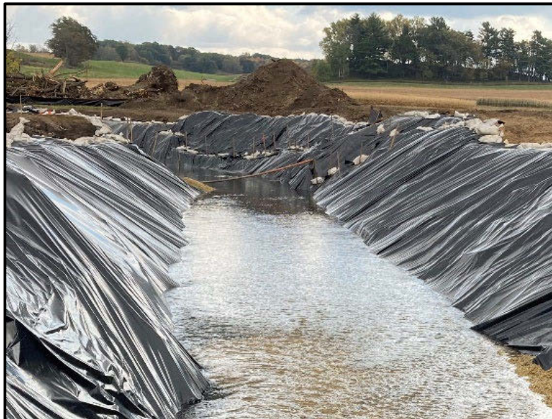
FIGURE 645-1 Polyethylene Sheeting Placement
