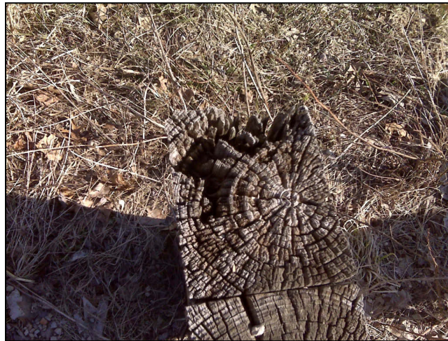
FIGURE 625-8 Rotten Posts
