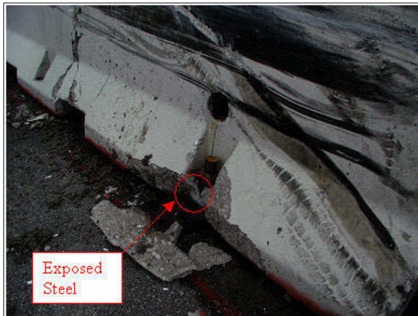
FIGURE 145-8 Anchor Hole Damage
