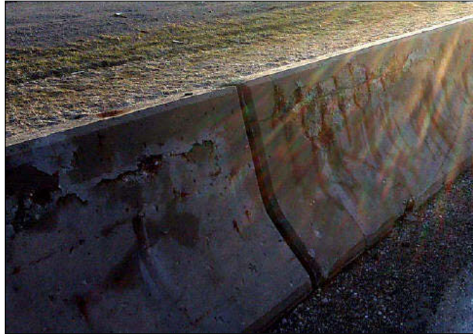
FIGURE 145-11 Exposed Steel Reinforcement
