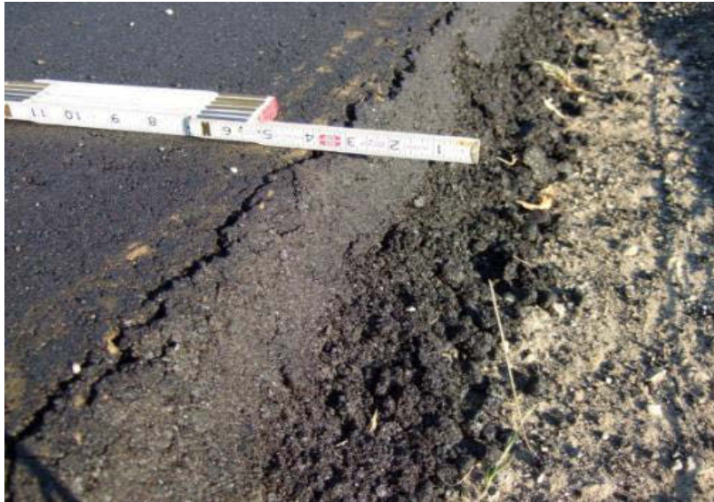
FIGURE 670-4 Cracked Edge
