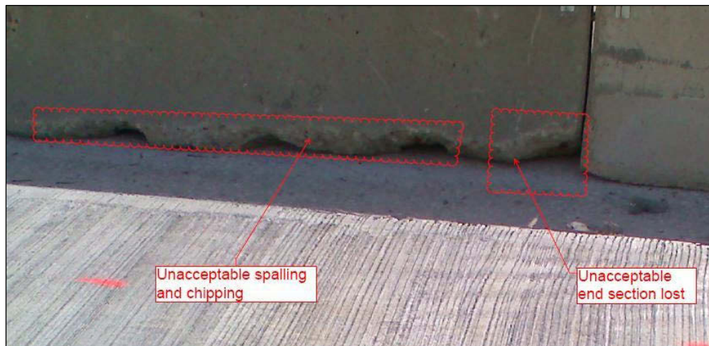
FIGURE 145-14 Spalling, Chipping, and End Section Loss
