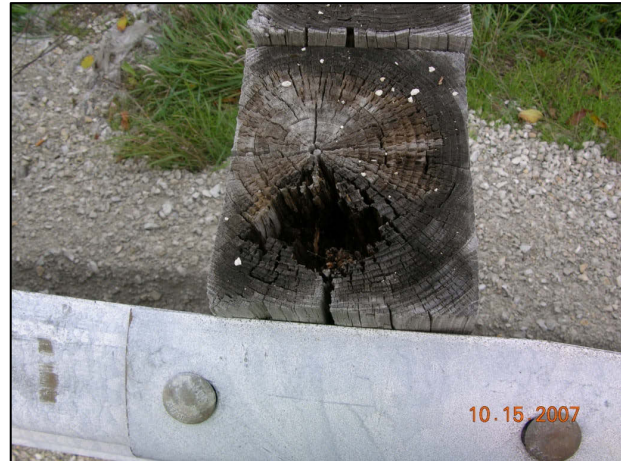
FIGURE 625-7 Rotten Block
