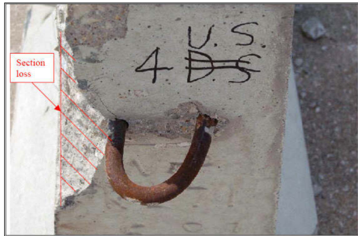
FIGURE 145-5 Loop Out of Alignment
