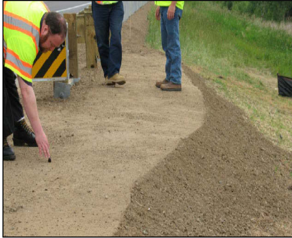
FIGURE 626-8 Marginal Grading
