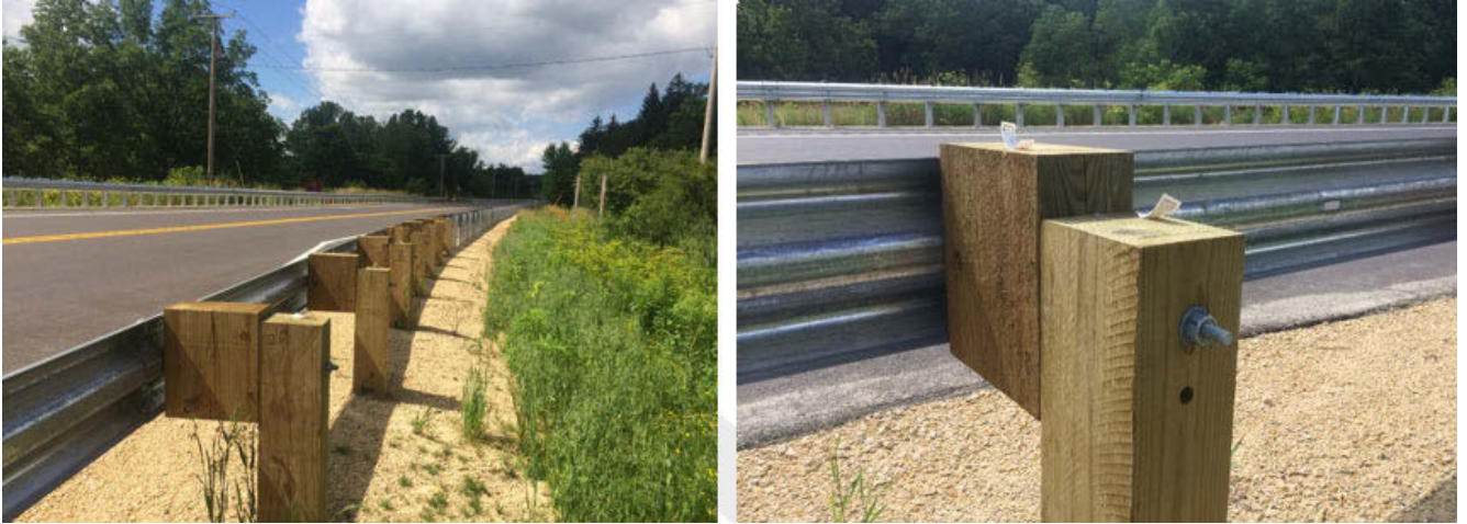
FIGURE 626-16 Block Height Adjustments
