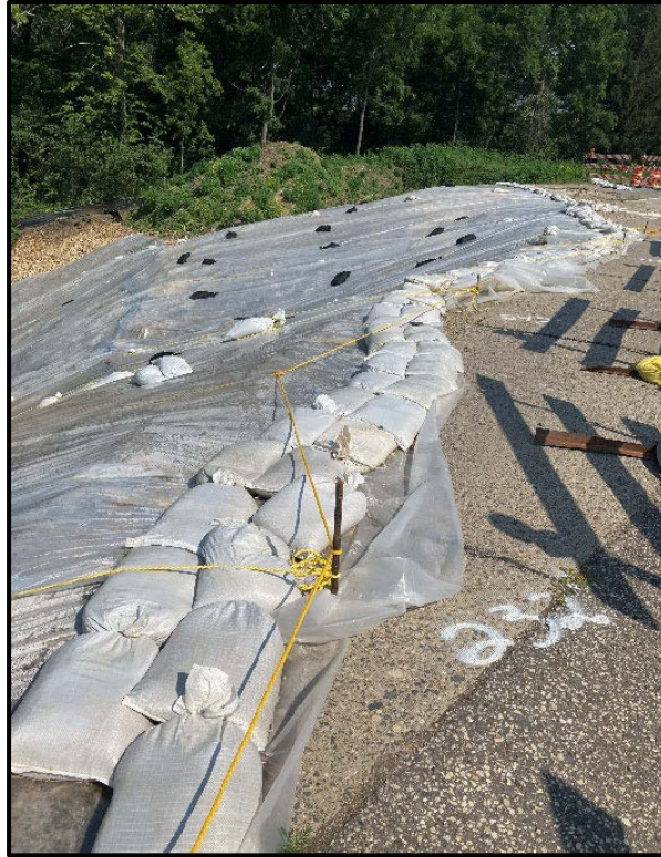
FIGURE 645-2 Securing Polyethylene Sheeting with Sand Bags
