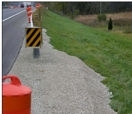
FIGURE 626-7 Marginal Grading
