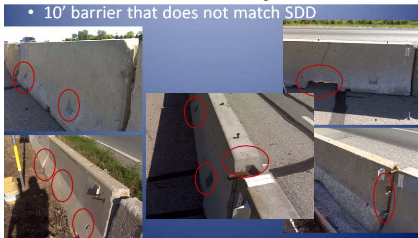
FIGURE 145-23 Barrier Not Matching Standard Details
