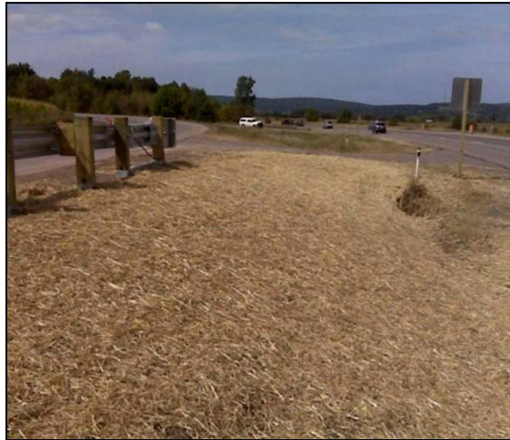
FIGURE 626-5 Desirable Grading
