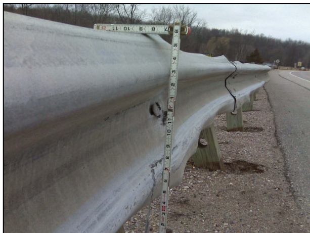
FIGURE 625-9 Rail Damage Examples Flattened Rail
