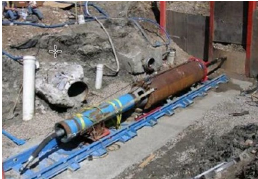
Figure 20.4 Pipe Ramming (Source AASHTO TC3)
