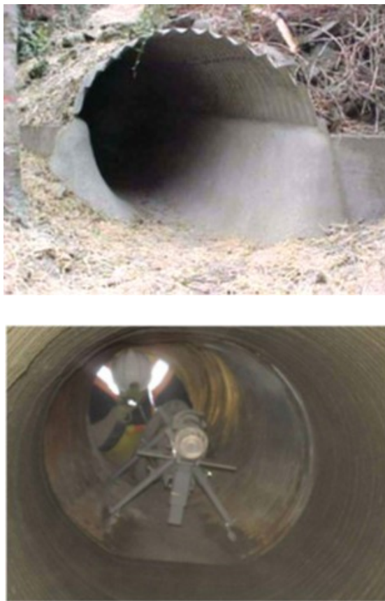
Figure 4.3 Spray-on Mortar Invert Repair and Cast Mortar Liner (Source FHWA and MNDOT)
