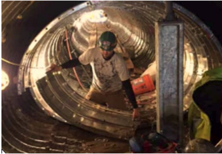
Figure 10.9 Liner Plate (Photo courtesy of Contech)
