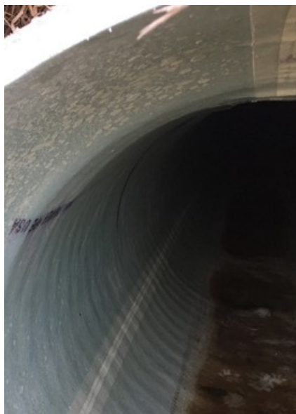
Figure 15.4 Roughness within CIPP Lined Culvert
