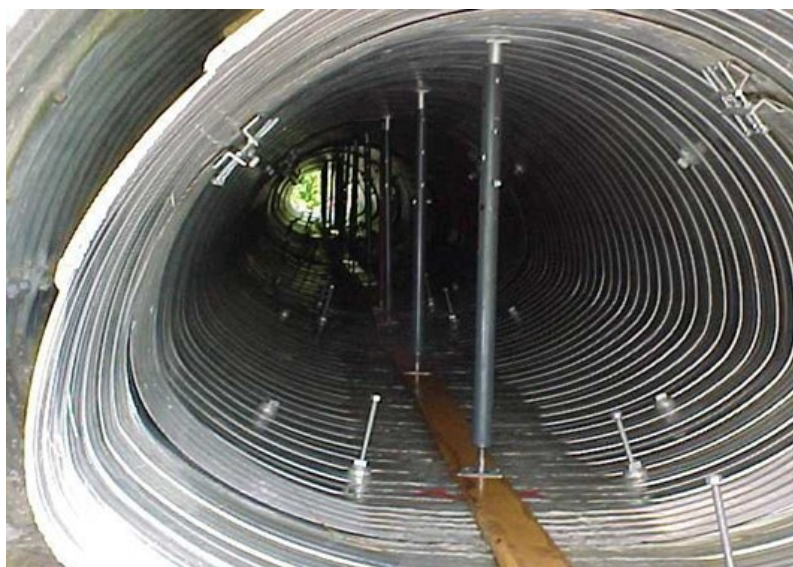
Figure 10.5 Floatation Bracing Examples with Blocking or Jacks (Photos courtesy of Contech)
