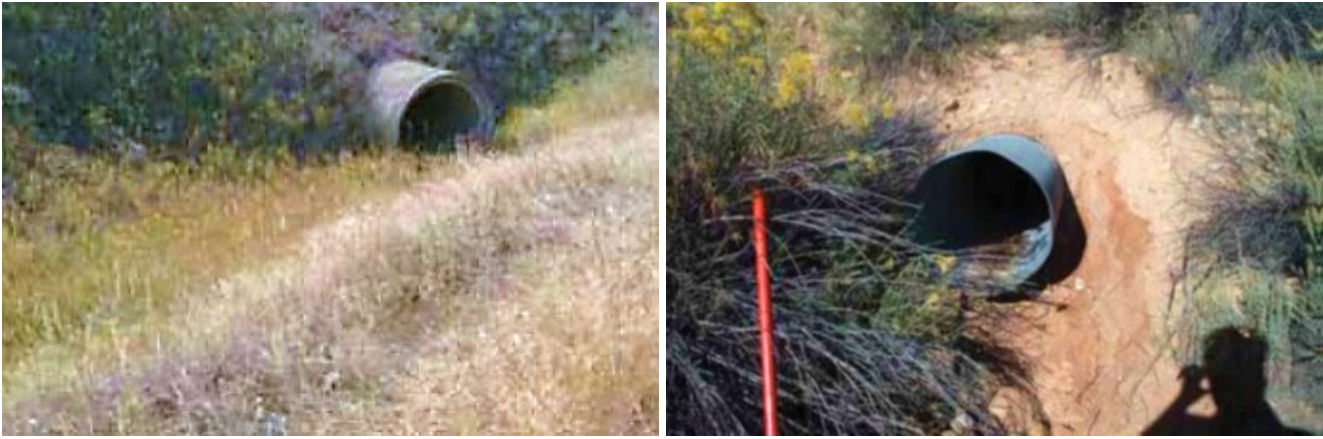
Figure 3.3 Stable and Unstable Channels Downstream of Culvert – Source FHWA and UDOT
