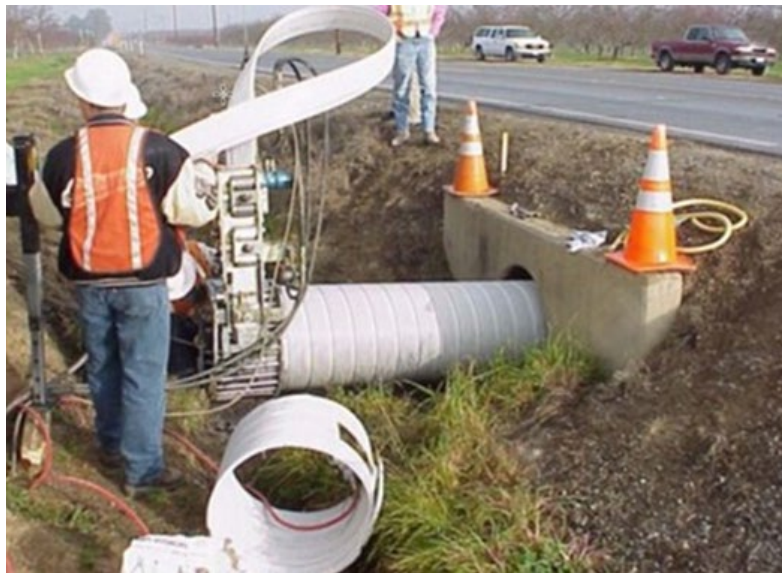
Figure 10.10 L Spiral Wound Liner (Photo courtesy of Caltrans, 2011)
