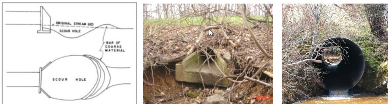
Figure 3.2 Scour Holes and Perched Culverts – Sources FHWA and WisDOT
