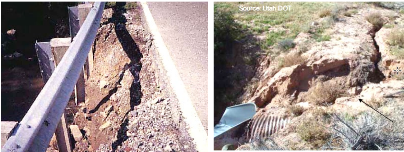
Figure 3.1 Erosion Damage to Downstream Embankment Slopes from Previous Overtopping - Sources FHWA and Utah DOT
