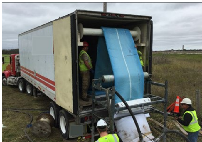
Figure 15.2 CIPP Culvert Lining
