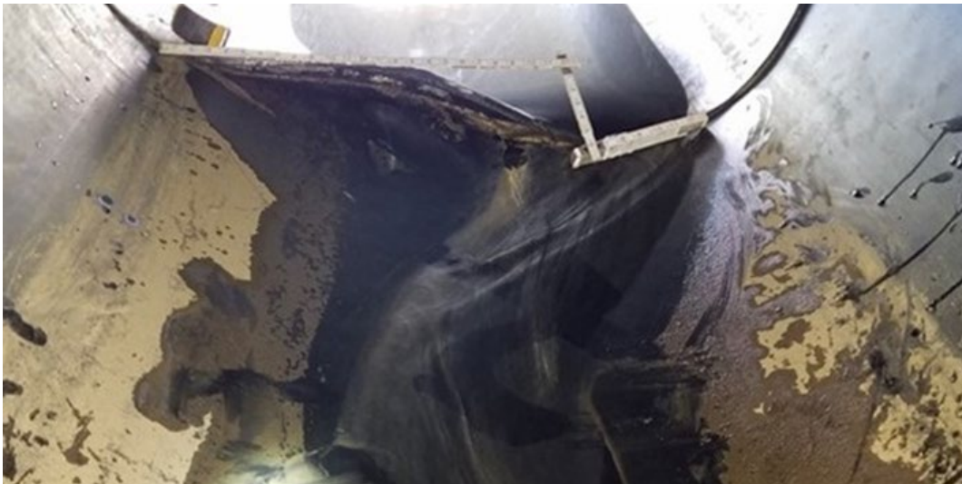
Figure 10.3 Bulge at Liner Joint Likely from Excessive Pumping Pressure
