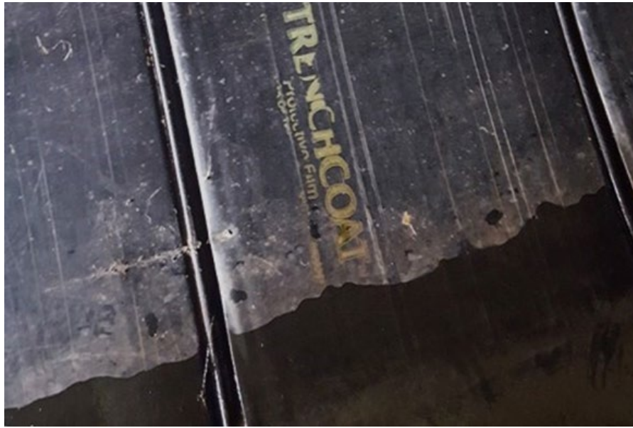
Figure 10.8 “Smooth” Polymer Coated CMP
