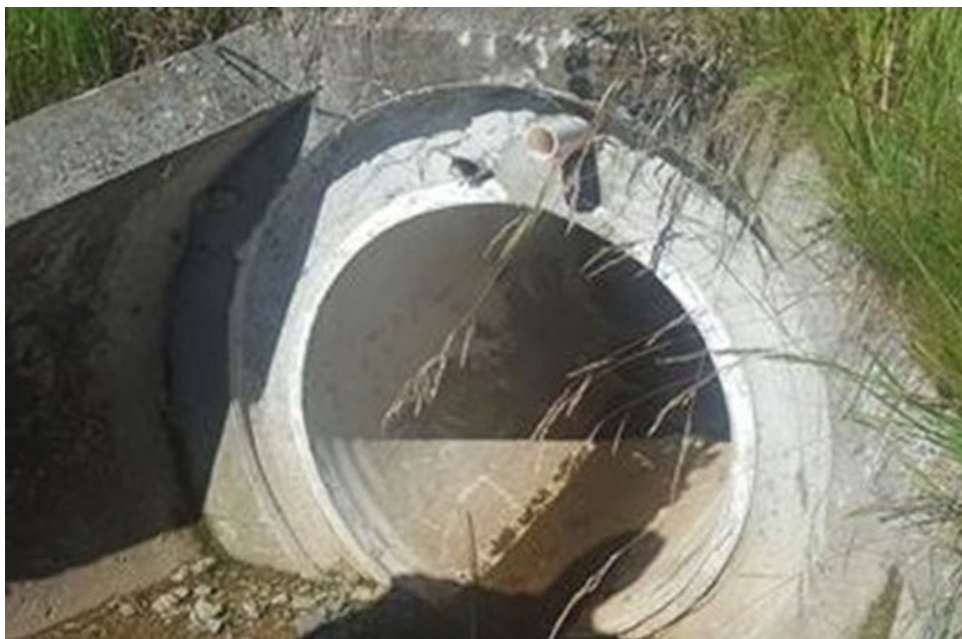
Figure 10.1 PVC Culvert Slipliner
