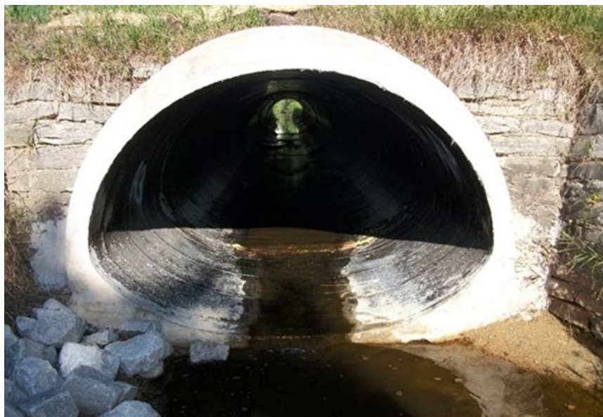
Figure 10.7 "Smooth-Lined" Poly-Coated CMP Arch used to Line Existing Steel Arch Culvert
