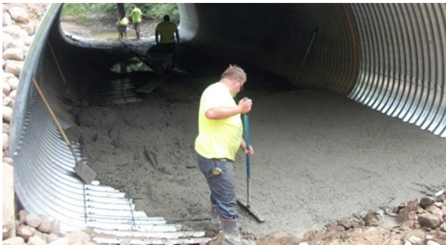
Figure 4.1 Extending and Invert Paving a Structural Plate Pipe Arch (Photo courtesy of Contech)
