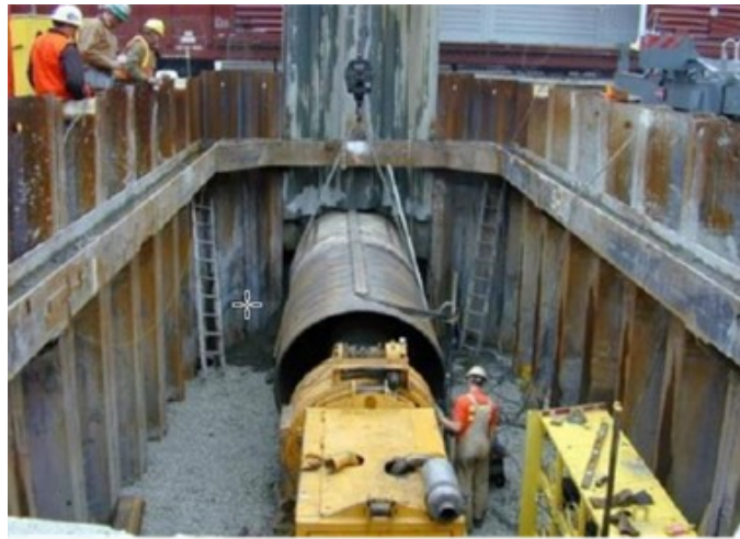
Figure 20.1 Jack and Bore Operations (Source AASHTO TC3)
