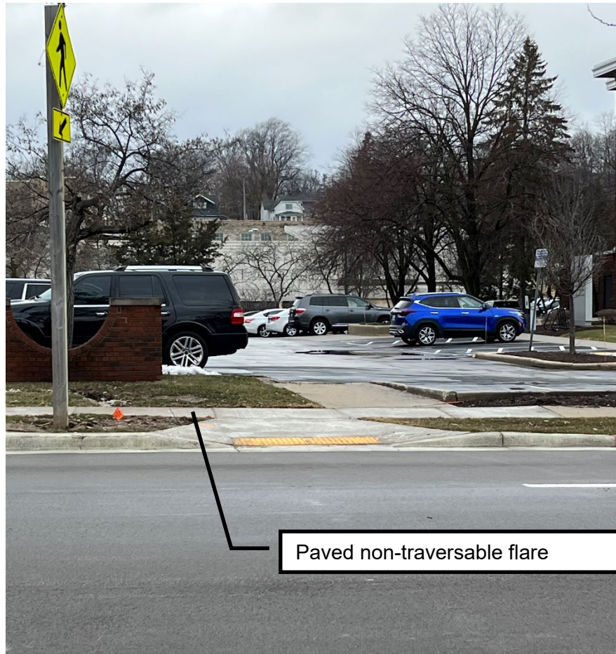
Figure 10.17 Paved non-traversable flares
