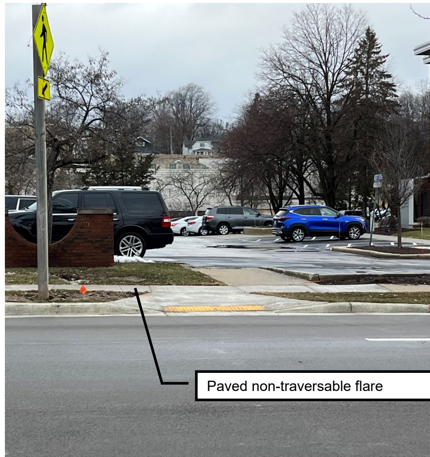
Figure 10.17 Paved non-traversable flares
