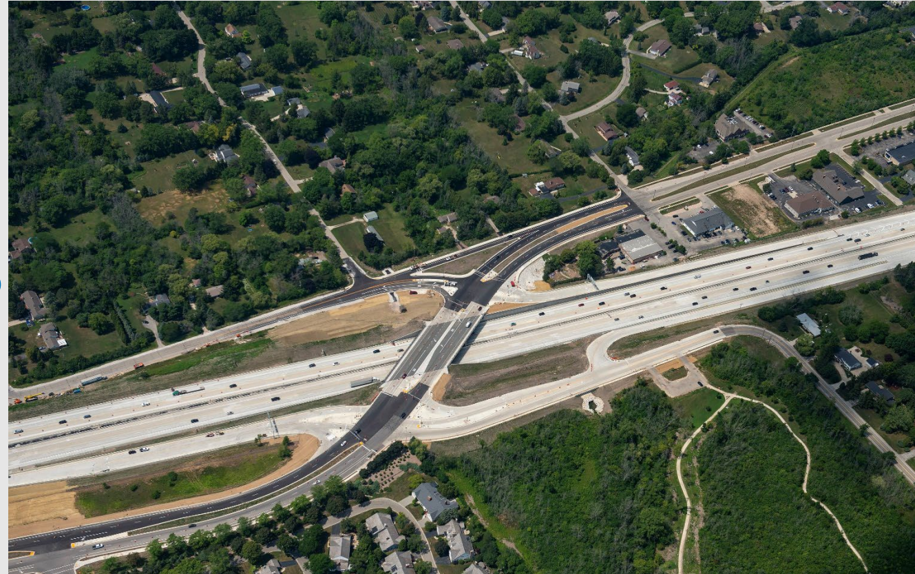
I-43, Port Washington Road Interchange, October 2023
