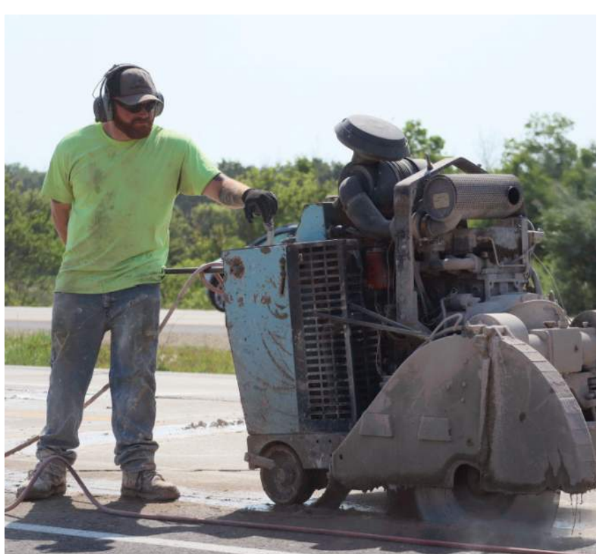
Dane County / US 18-151 Hard Rock Sawing & Drilling Specialist Co.
