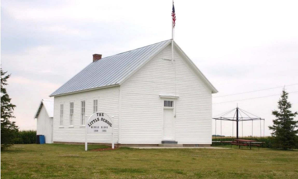
Example of a one-room schoolhouse in La Crosse County in which interior access was completed for the Section 106 compliance survey.
