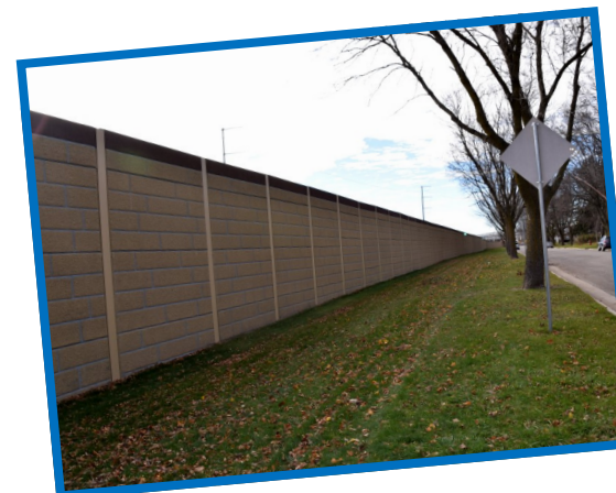
Noise barrier on residential side.
