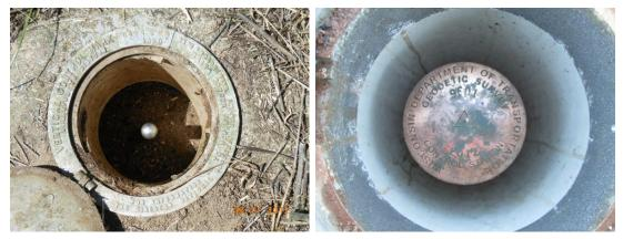
c. A Stainless Steel Rod Geodetic Survey Control Station is either surrounded by white plastic witness posts (vertical only) or orange 4"x4" guard posts (horizontal & vertical), depending on the survey accuracy of the control point.
