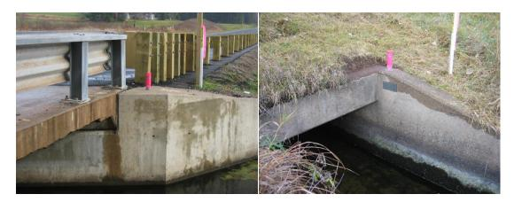
c. Whenever possible, a Bronze Survey Disk set in a concrete structure is marked with a single white witness post (Vertical control point).
