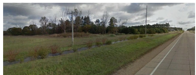
Figure 2: LSF along WIS 82 east of Oxford
