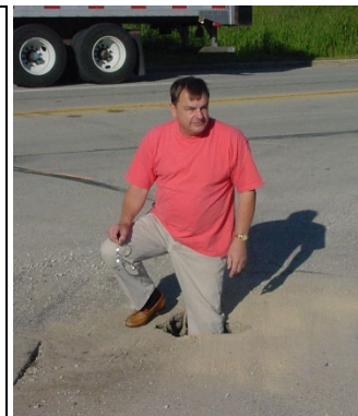
Figure 3: Improper pothole restoration
