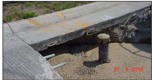
Figure 2: Concrete pavement repair without sawcut. Note top of pavement edge and missing dowel bar. In lower picture, dowel bars in gutter are bent and not ready to accept slurry.
