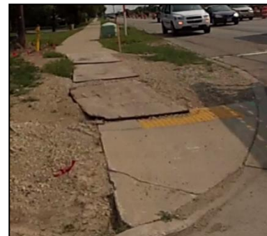
Figure 1: Sidewalk work not meeting ADA requirements
