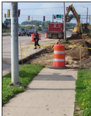
Figure 1: Sidewalk work not meeting ADA requirements
