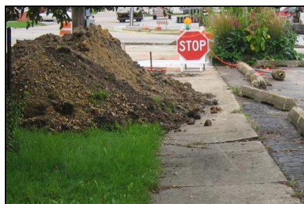
Figure 2: Sidewalks blocked by vehicles, materials, signs, and devices
