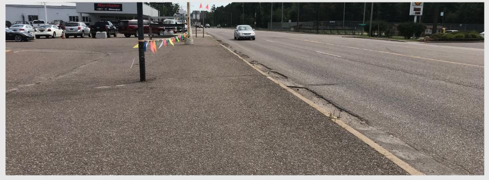
The existing pavement is deteriorating, rutting, and cracking
