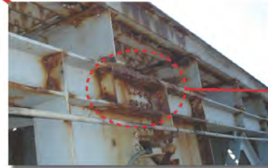
Clean & Paint Structural Steel
