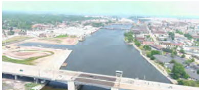
Photo of Mason Street Bridge from June 19, 2023
