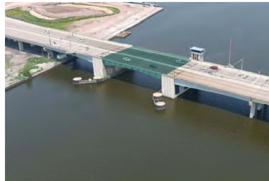
The bascule portion of the bridge in a lowered position (shown shaded green).
