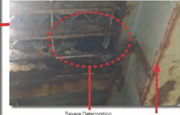
Corroded Stringer
