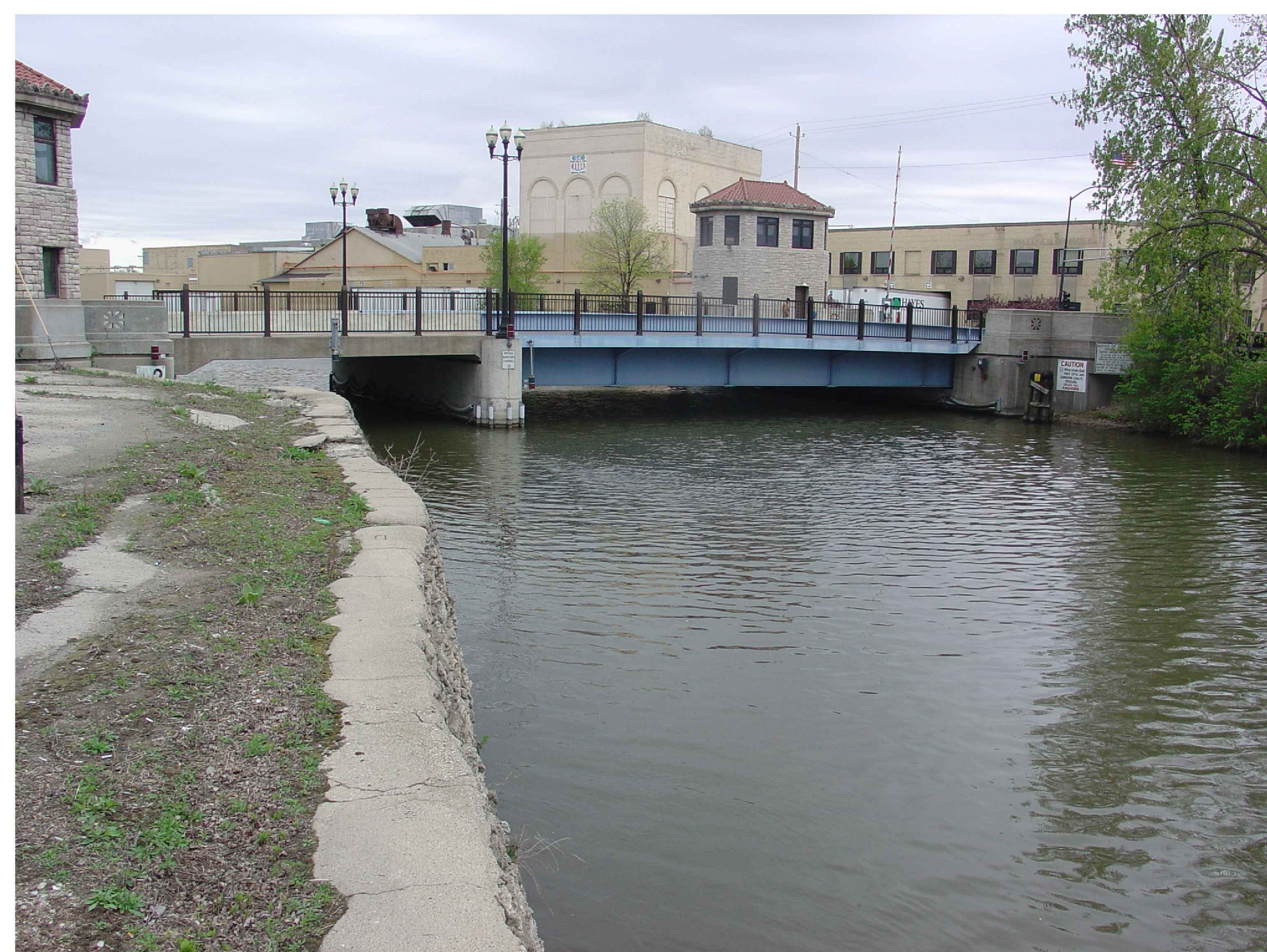
TAYCO STREET BRIDGE AUXILIARY SPAN
