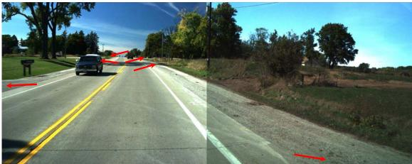
Respondents identified access along the two-lane section of WIS 21 as a concern. This segment, just west of Leonard Point Road, shows the location of six separate driveways with direct access to/from WIS 21 within less than one-quarter mile. The driveway access points are indicated by the arrows.
