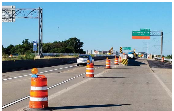
Example of a construction lane closure
