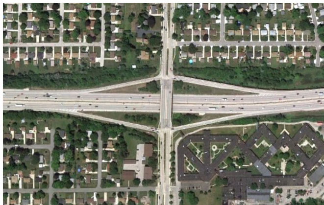
Example of typical urban service interchange (Interstate 43 [I-43]/Interstate 894 [I-894] at 60 th Street)
