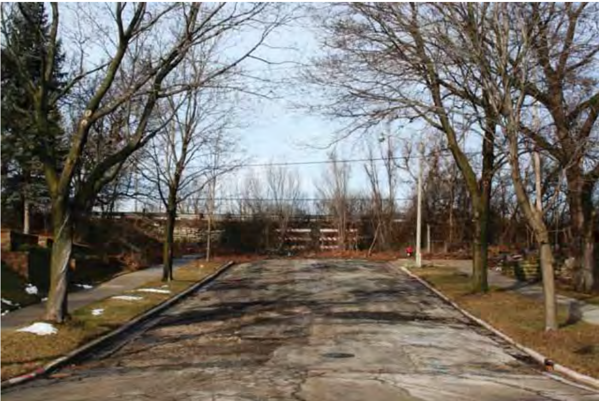
Exhibit A-7: Location 5 (Landscape Unit 1) From S. 61 st Street north of W. Dixon Street looking north at the end of the street adjacent to I-94.
