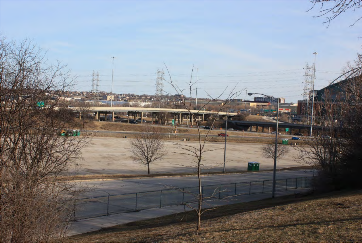
Existing Condition: From N. Story Parkway looking southeast over Yount Drive towards the US 41/I-94 interchange, Miller Park parking areas, and the northeastern edge of Miller Park.
