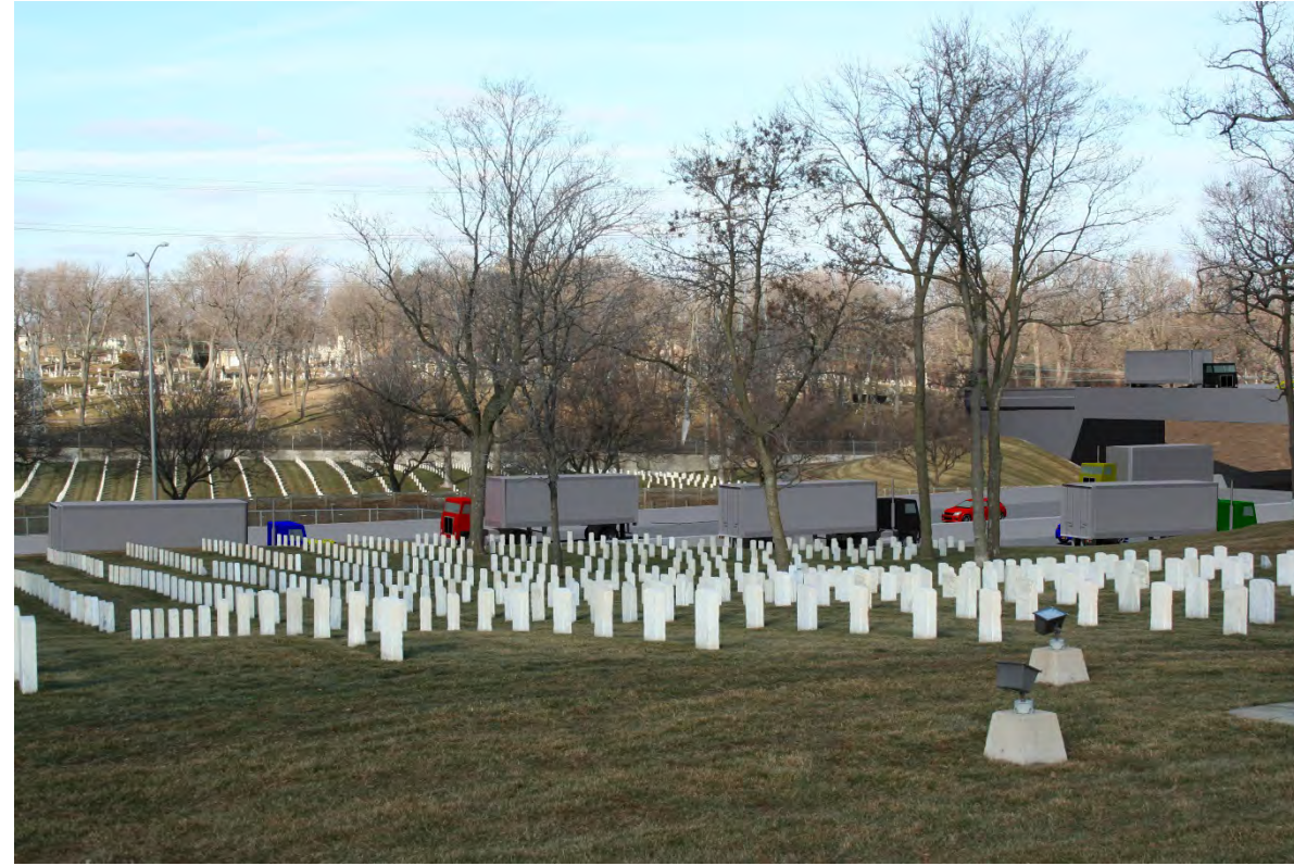
Simulation E: Modified Alternative C2 (At Grade) with connection to VA from Mitchell Boulevard south of I-94.
