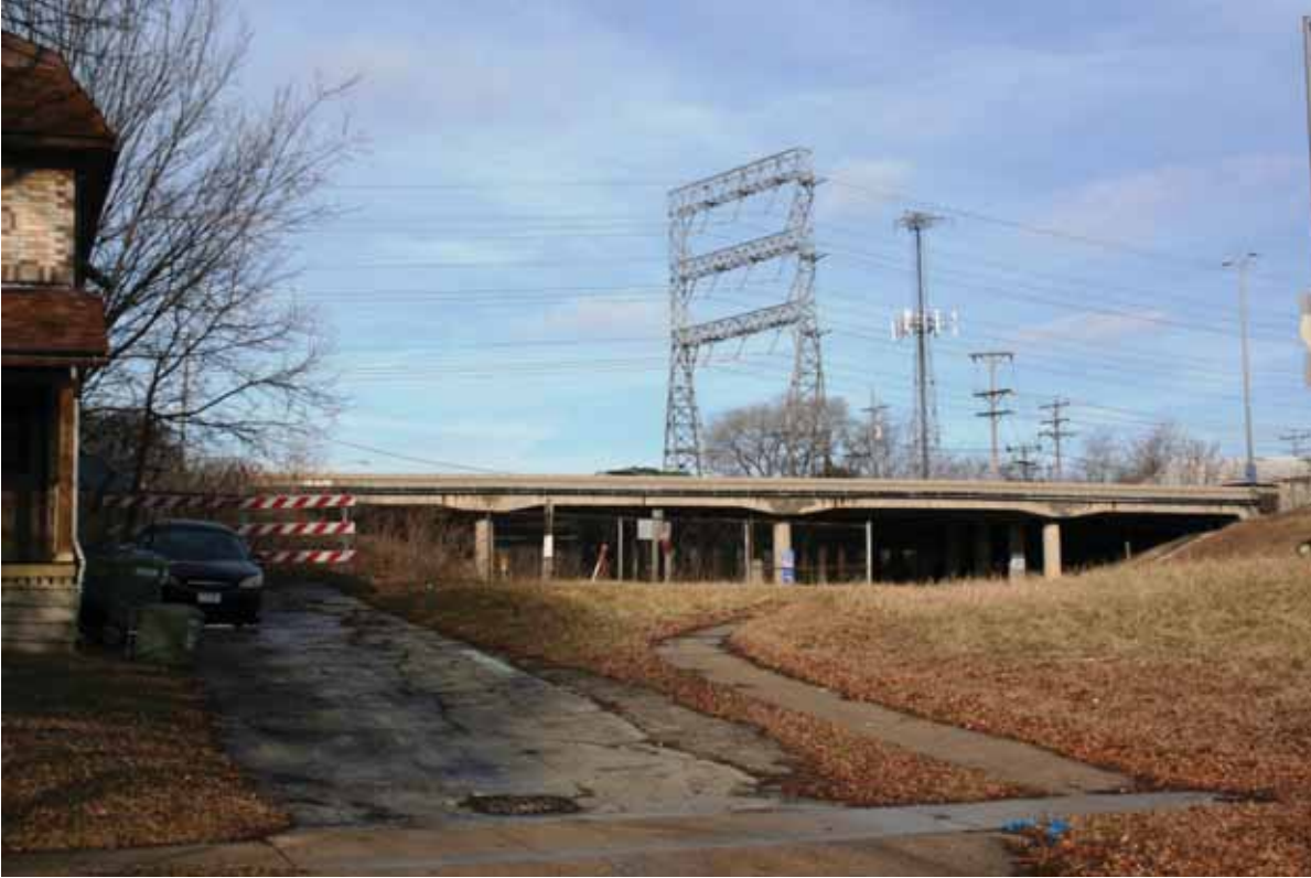
Existing Condition: From Dixon Street west of Hawley Road looking northeast at I-94 overpass.
