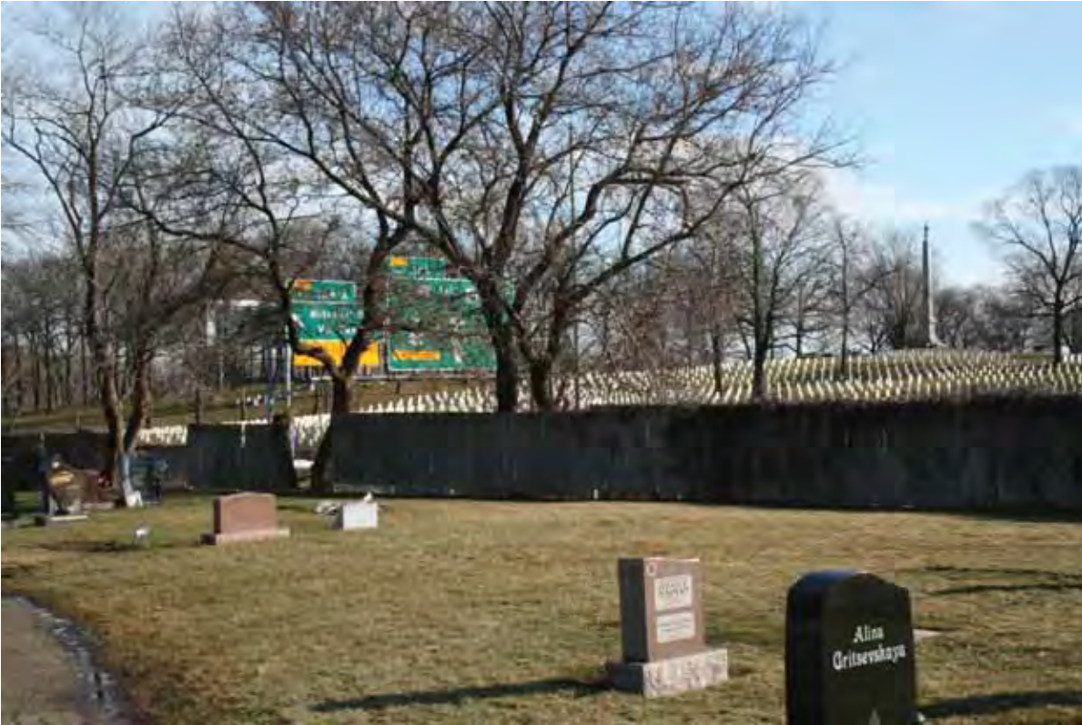
Existing Condition: From east end of Beth Hamedrosh Hagodol Cemetery looking southeast at fence screening view of I-94 freeway lanes and main part of Wood National Cemetery.
