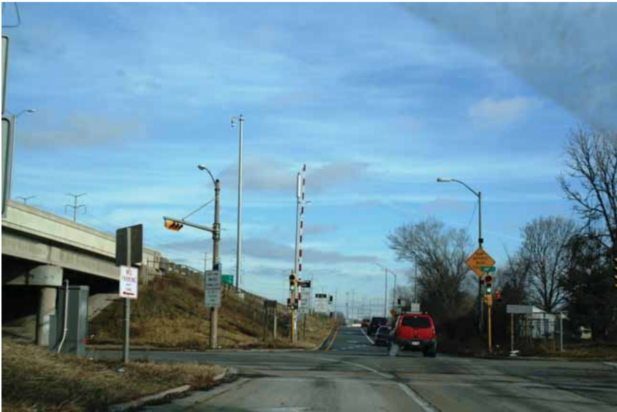
Exhibit A-3: Location 1 (Landscape Unit 1) From eastbound W. Kearny Street just west of S. 68 th Street looking east at I-94 overpass over S. 68 th Street and the east-bound onramp to I-94.
