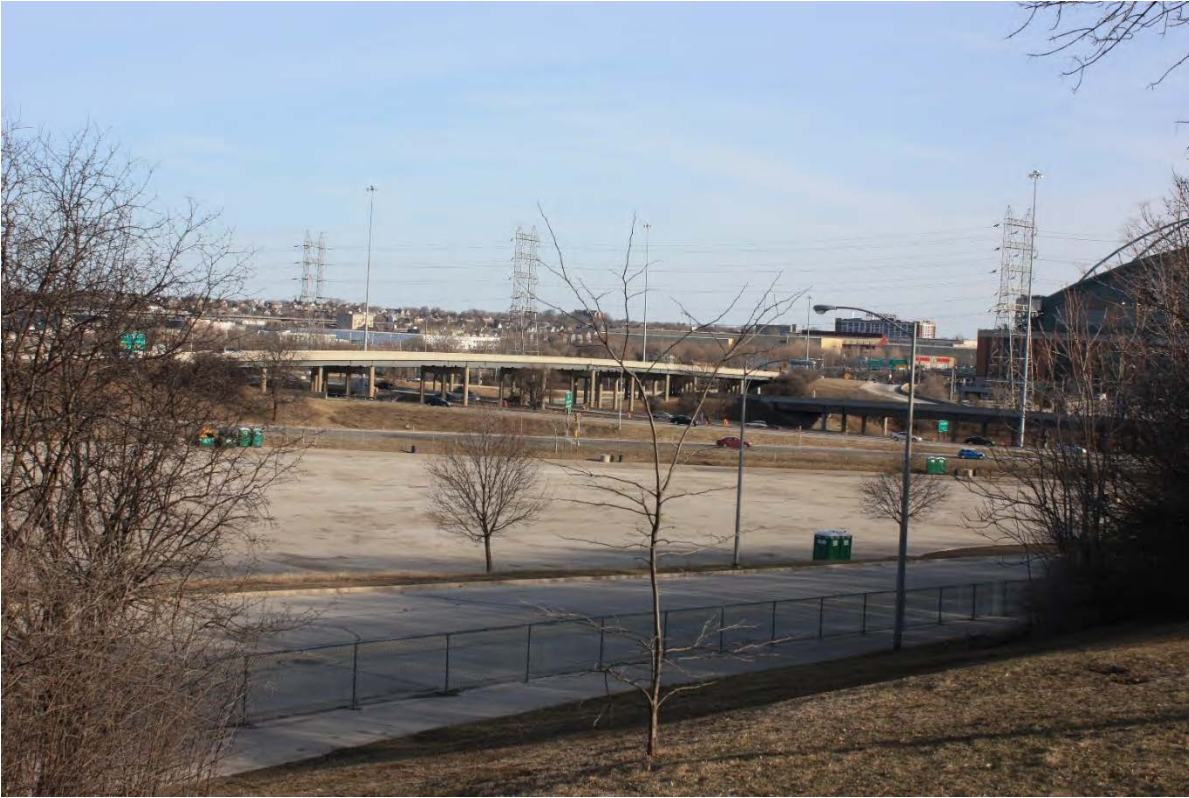
Existing Condition: From N. Story Parkway looking southeast over Yount Drive towards the US 41/I-94 interchange, Miller Park parking areas, and the northeastern edge of Miller Park.
