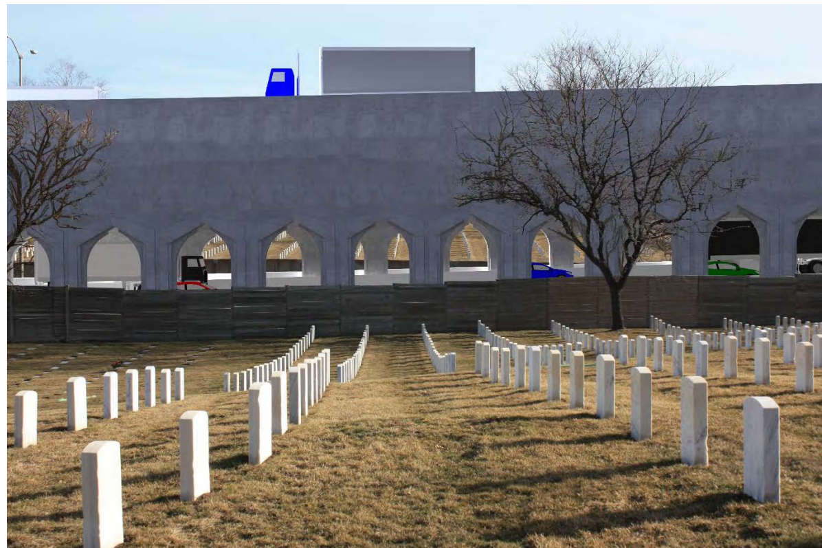
Simulation C: Modified Alternative C5 (Double-Deck) with All Up option and openings on the lower deck.
