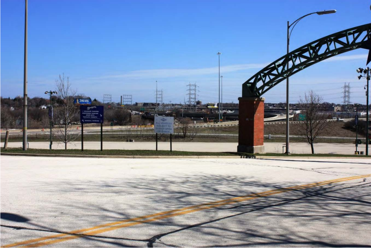
Existing Condition: From Yount Drive (just east of Story Parkway) looking southeast towards entrance to Miller Park, parking areas, and the I-94/US 41 interchange.
