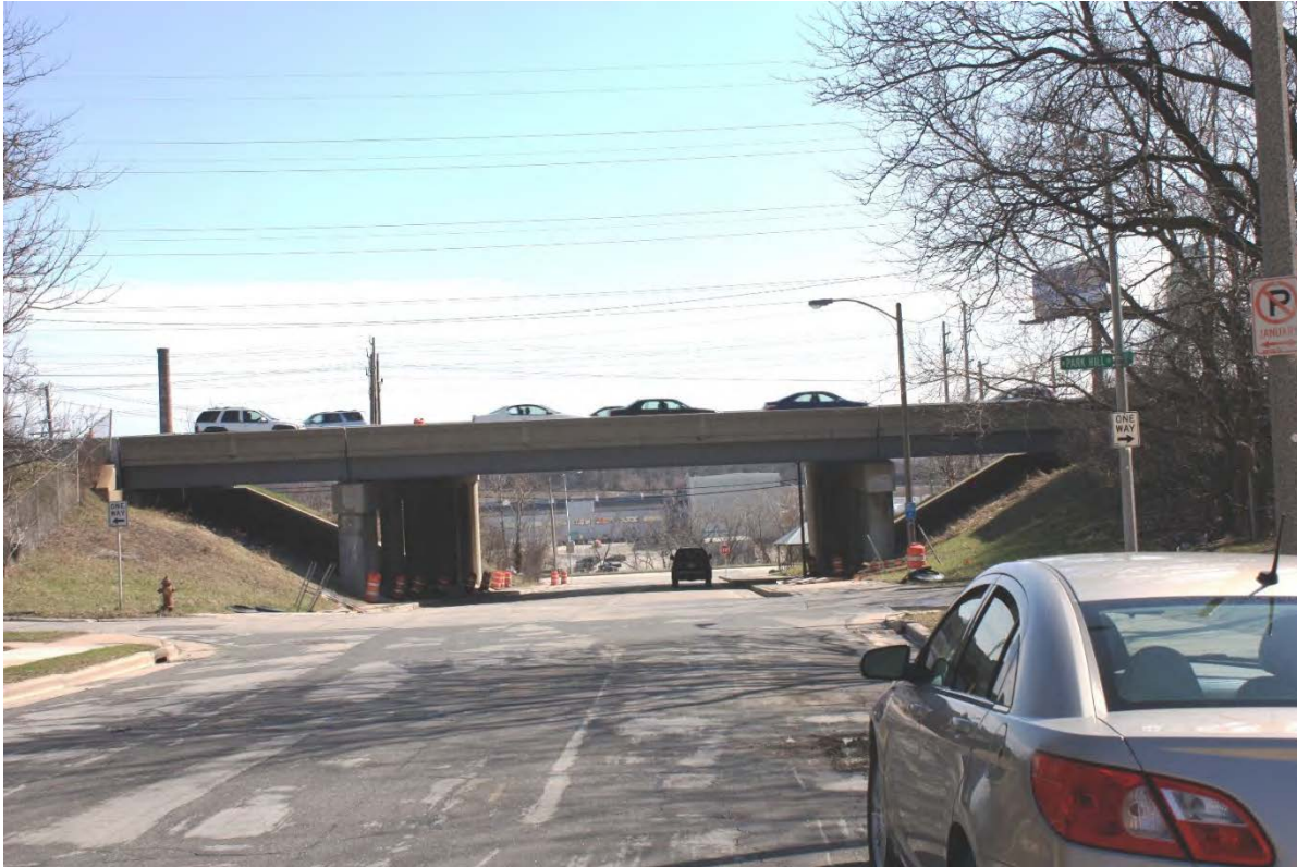
Existing Condition: From 32 nd Street north of Park Hill Avenue looking south at I-94 overpass.
