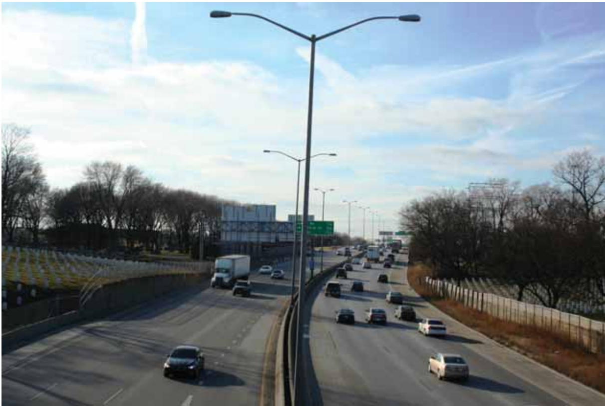
Exhibit A-13: Location 11 (Landscape Unit 2) From Zablocki Drive bridge over I-94 looking west over I-94. Note the main part of Wood National Cemetery on left (south) side of I-94 and the north parcel on the right (north) side.
