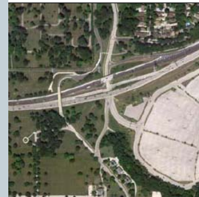
Mitchell Boulevard Interchange
