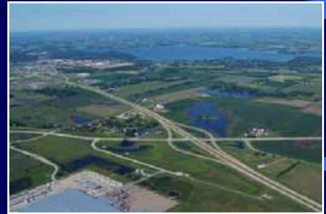
County A Interchange
