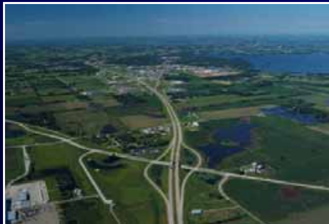
County A Interchange
