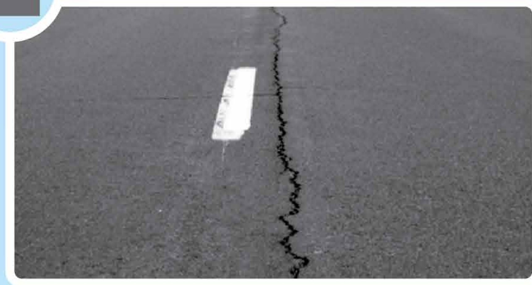
Cracking of the asphalt overlay causes deterioration of the bridge deck.
