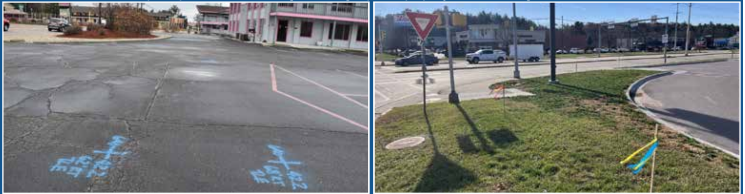
Example of paint and lath markings showing impacted property locations along the US 12 corridor.
