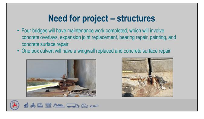
The bridges and box culverts were originally constructed in 1969. Some along this section of US 14 require routine maintenance to maintain their function.
