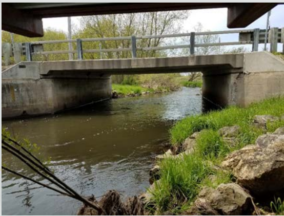
East Bridge Face
