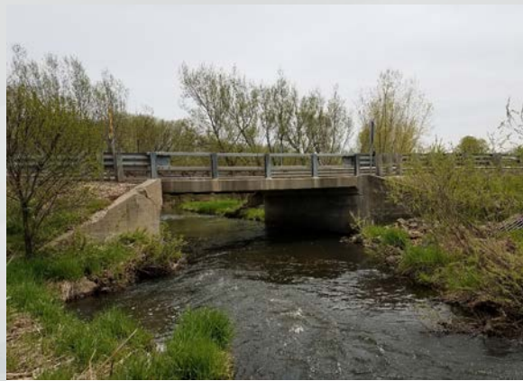
West Bridge Face
