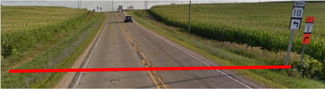
Culvert pipe 0.10 miles south of County Highway V
