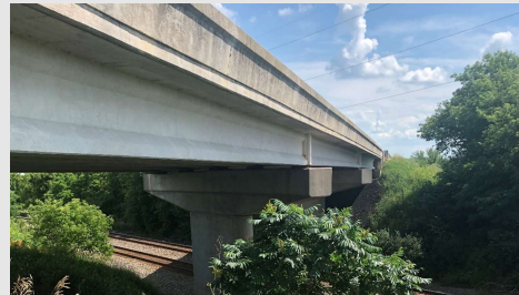
Bridge (B-11-27) over railroad
