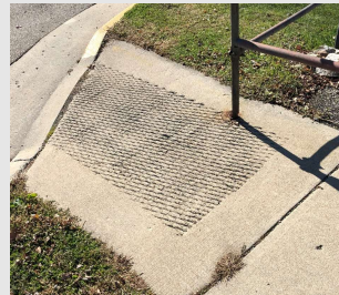
2 nd St northwest curb ramp
