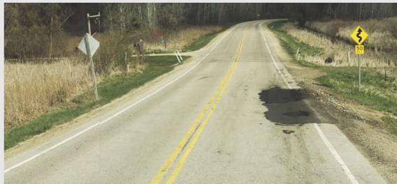
Existing pavement on WIS 146
