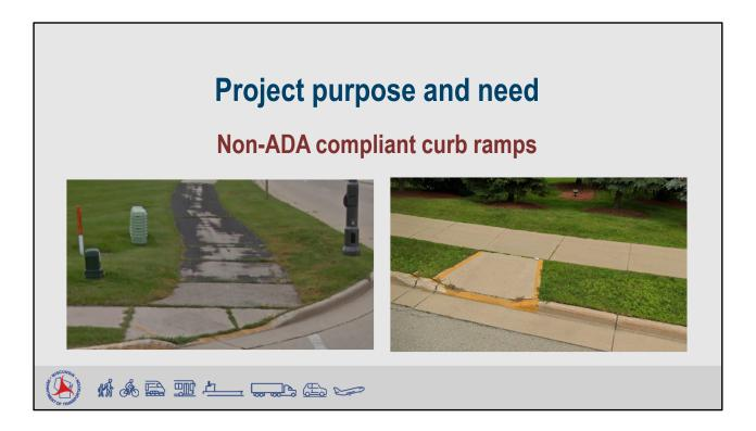
In addition to the roadway, Highway 19 has curb ramps within Sun Prairie City limits that are not in compliance with the current Americans with Disabilities Act (ADA) standards and must be upgraded to be within compliance. Pedestrian access will be always maintained on one side Highway 19 during the curb ramp upgrades.
