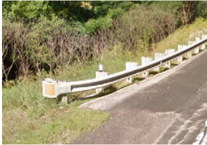
Existing WIS21 Guardrail
