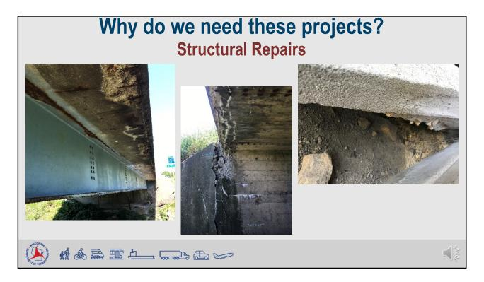
The northern project also has improvement needs on two existing structures. The bridge over Rountree Branch, just south of Business 151 in Platteville, has several areas of damaged concrete. Significant erosion is also occurring under the structure at the abutments. In addition, a box culvert near the Blockhouse Road intersection has damaged concrete and exposed rebar.
