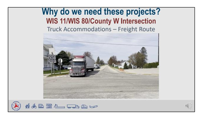
This video shows a typical semi traveling Eastbound to Northbound through the intersection. Notice how the semi is forced to overtrack into the opposing Southbound lane in order to complete the movement.
