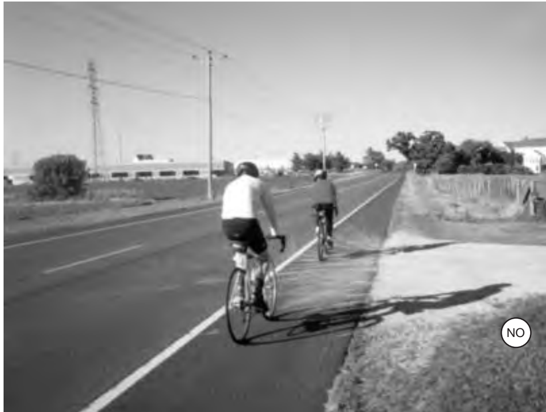
Figure 2-10 (above): Bad pavement edges create hazards for bicyclists.
