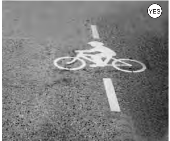
Figure 2-52: Close-up of Madison-style loop detector pavement marking.
