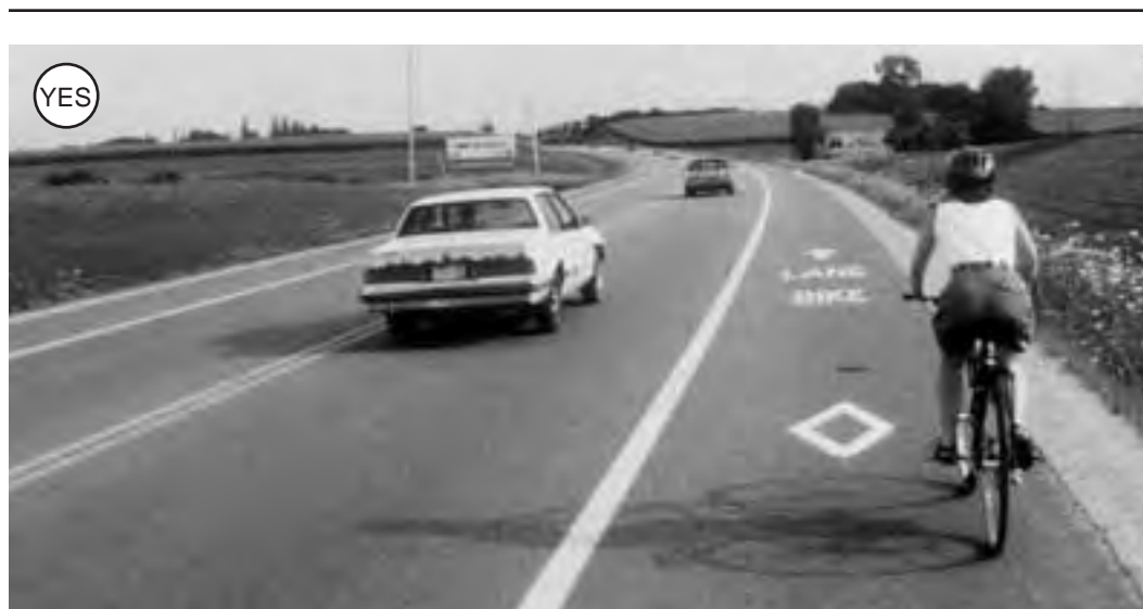
Figure 2-32: Adequate paved shoulders on rural roads provide clearance between bicyclists and passing motorists. In this particular instance, the shoulder is marked as a bike lane, since it links a state park entrance and a state trail.
