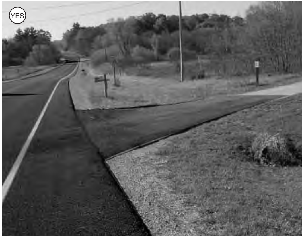
Figure 2-36: Paving into gravel driveways or side roads, or in this case a stone- surfaced state trail, can help keep debris from covering the paved shoulder.
