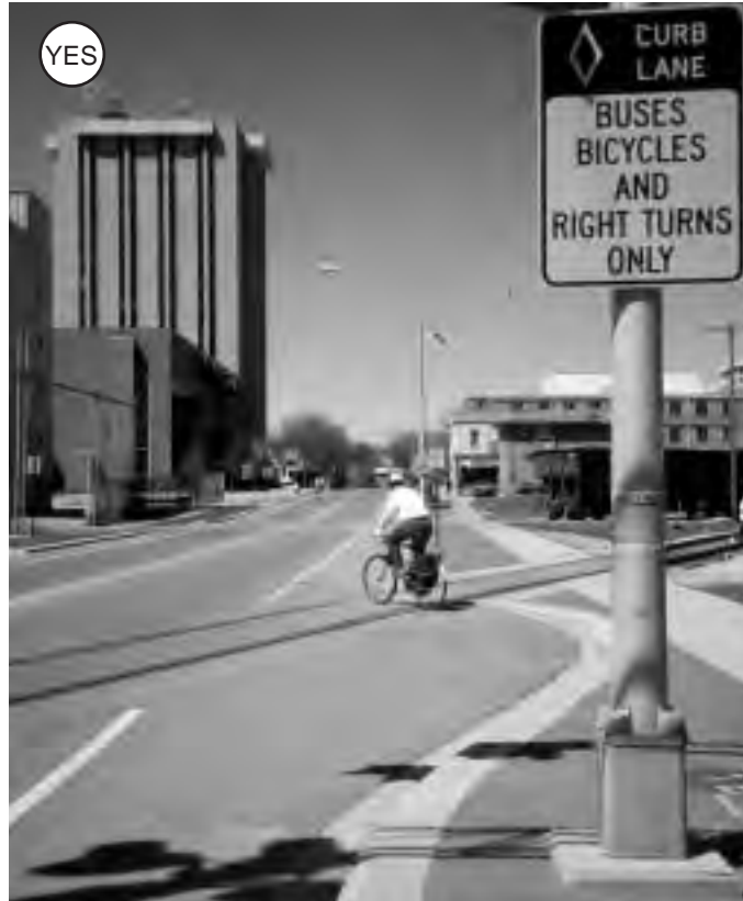
Fig. 2-43: A flared approach provides a safer angle for bicyclists crossing a diagonal railroad track.
