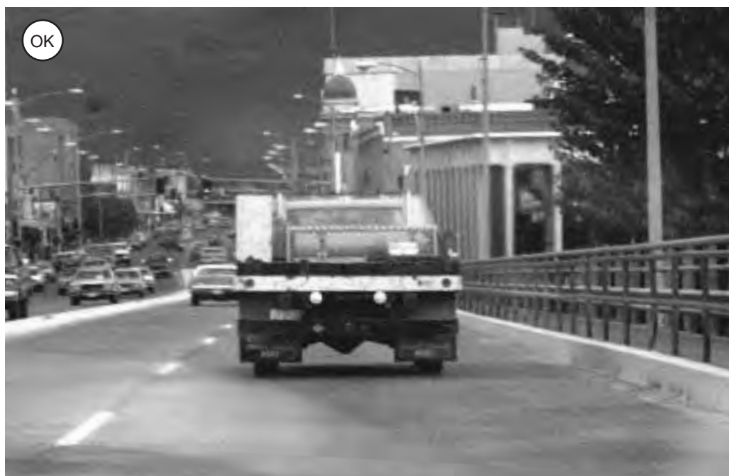
Figure 2-54: Lane striping was shifted to the left on this 4-lane downtown bridge to give 15-foot outside lanes and 11-ft. inside lanes.
