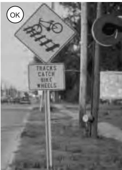
Fig. 2-44: Warning sign W11-59.3 (similar to that shown) may be used where the hazard cannot be completely eliminated.
