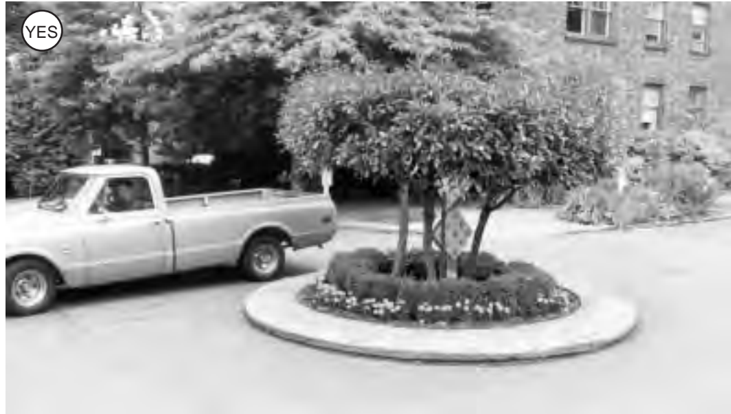
Figure 2-64: A residential street traffic circle slows traffic at intersections and reduces the frequency of intersection crashes.
