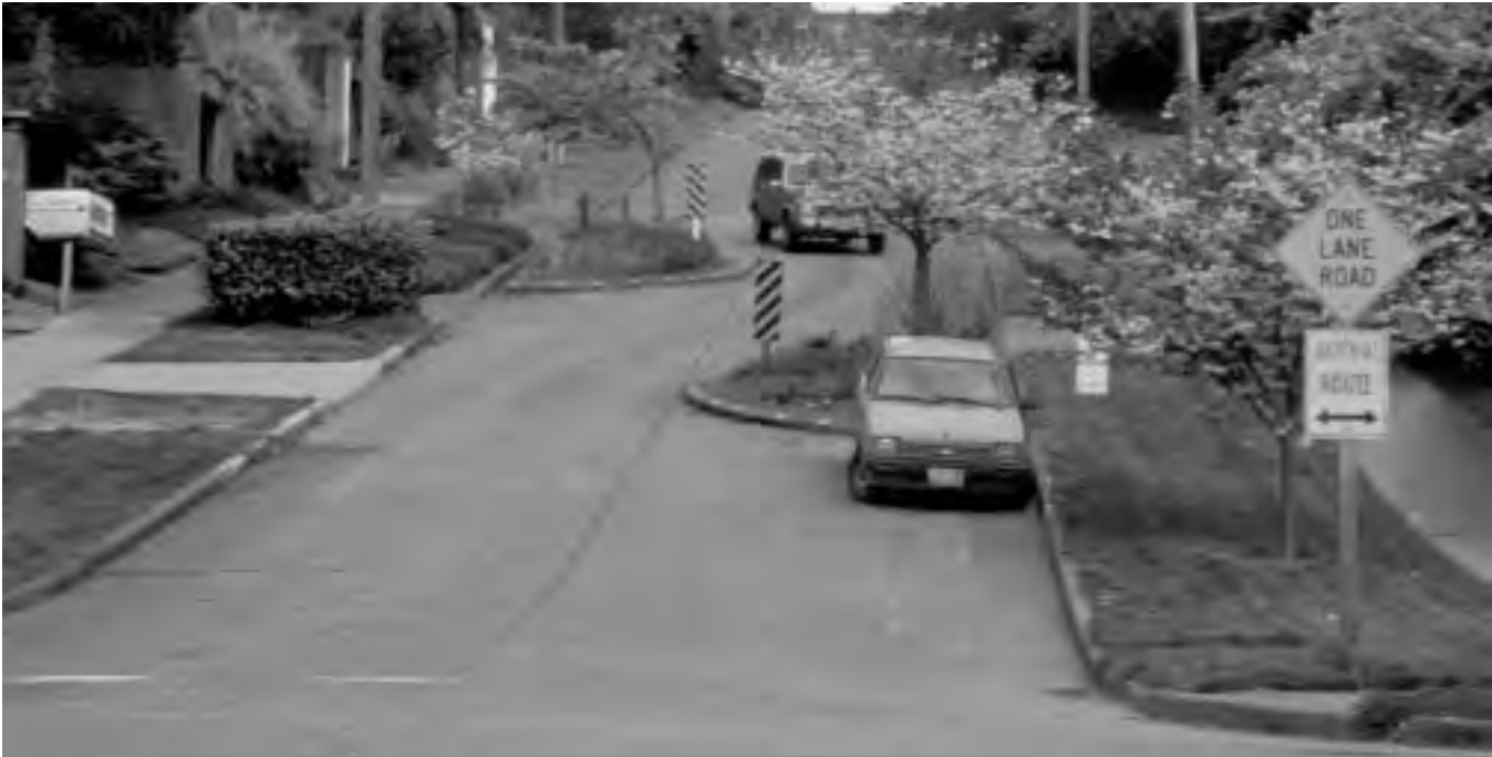
Figure 2-75: A chicane forces traffic to divert left and then right.
