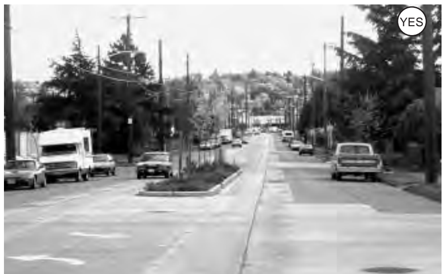
Figure 2-31: Designers replaced 4 through lanes on this narrow road with 2 through lanes, a center turn lane, and space for bicyclists.
