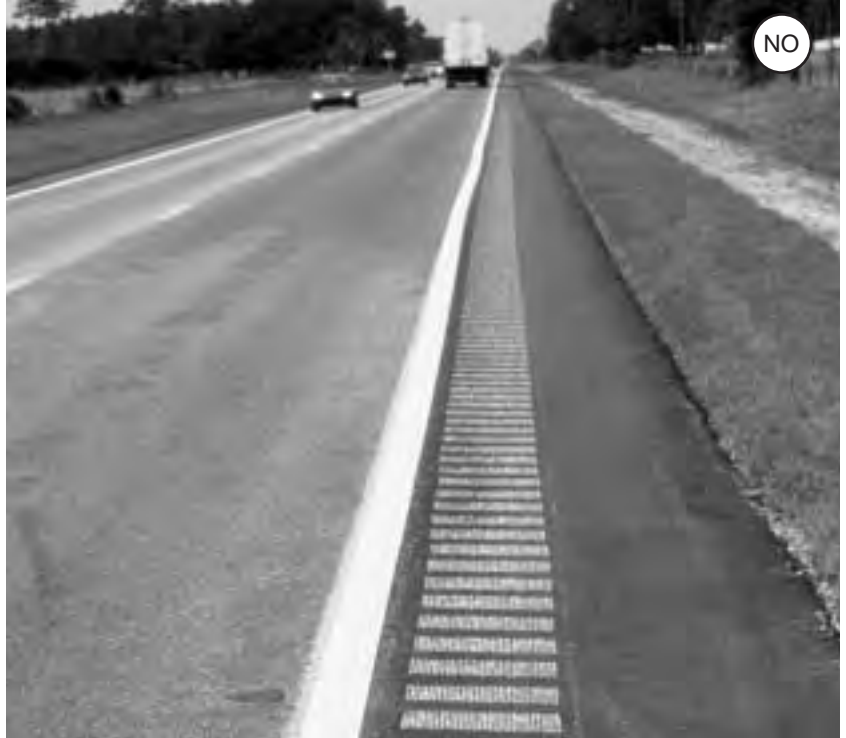
Figure 2-37: Continuous shoulder rumble strips provide an unsafe surface for bicycling. Gaps every 40-60 ft. that are 12 ft. long should be provided for bicyclists to safely move between the shoulder and travel lane as necessary to avoid debris, make turns, pass, etc.
