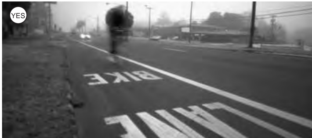
Figure 3-31: Lane markings should be spaced about every 600 ft. (180m) for urban sections and every 1 mi. (1.6km) for rural sections.
