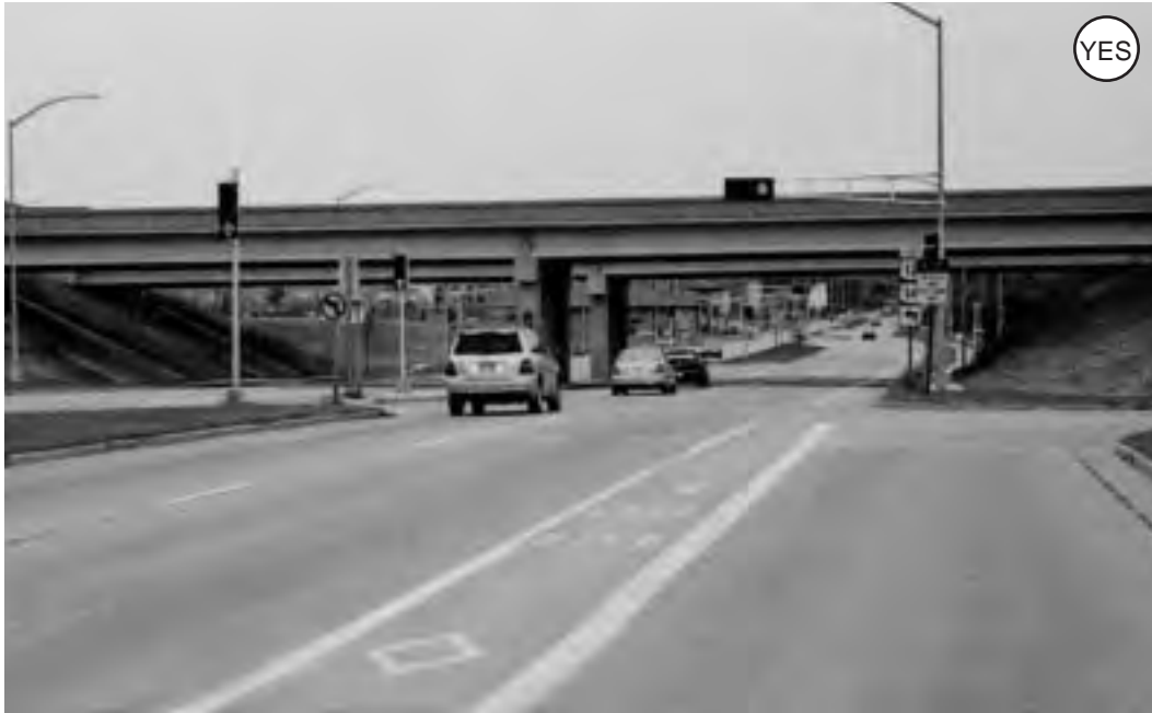
Figure 3-44: An urban-style interchange design is easier for bicyclists to negotiate than a rural-style design with its high-speed merges and broad sweeping curves.
