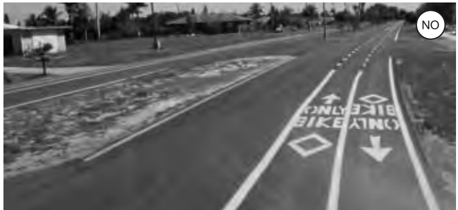
Fig. 3-3: Two-way bike lanes make it harder for bicyclists and motorists to see each other and increase conflicts at intersections and driveways.
