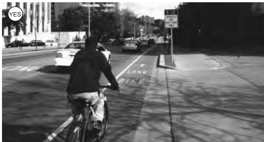
Fig. 3-1: A typical striped bicycle lane on a section of roadway without parking.
