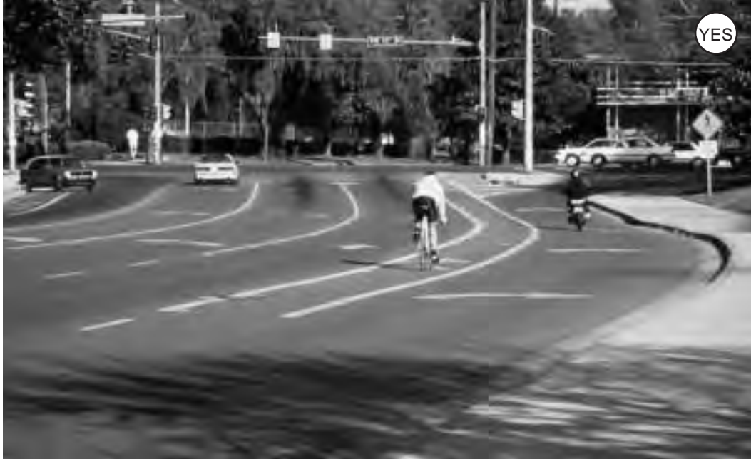
Figure 3-33: Well-designed intersection bicycle lanes can help bicyclists deal with the complexities of traffic movements.
