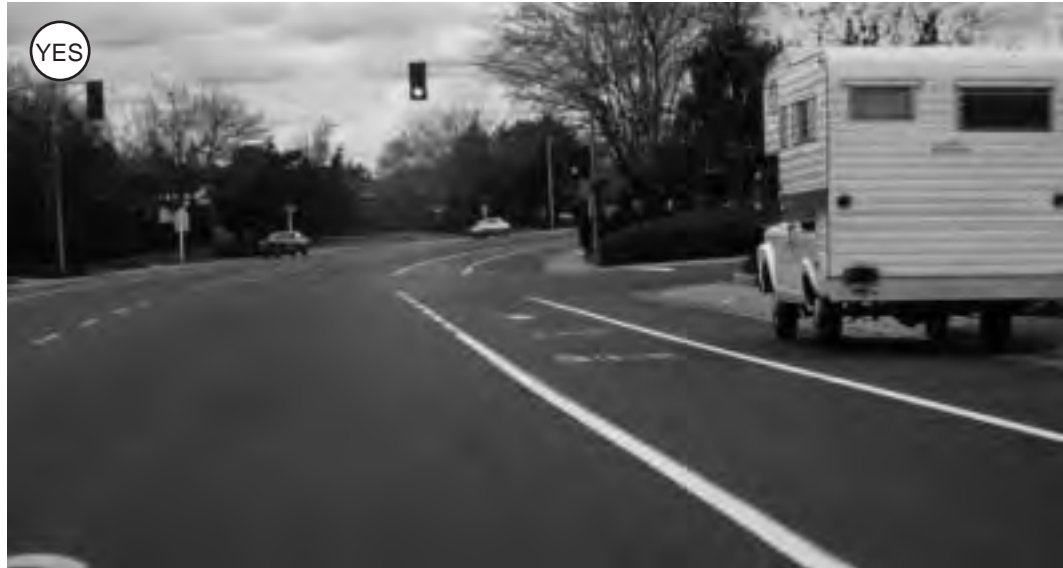
Fig. 3-4: The proper location for a bicycle lane is to the left of the parking lane. In this location, bicyclists and motorists can clearly see each other.
