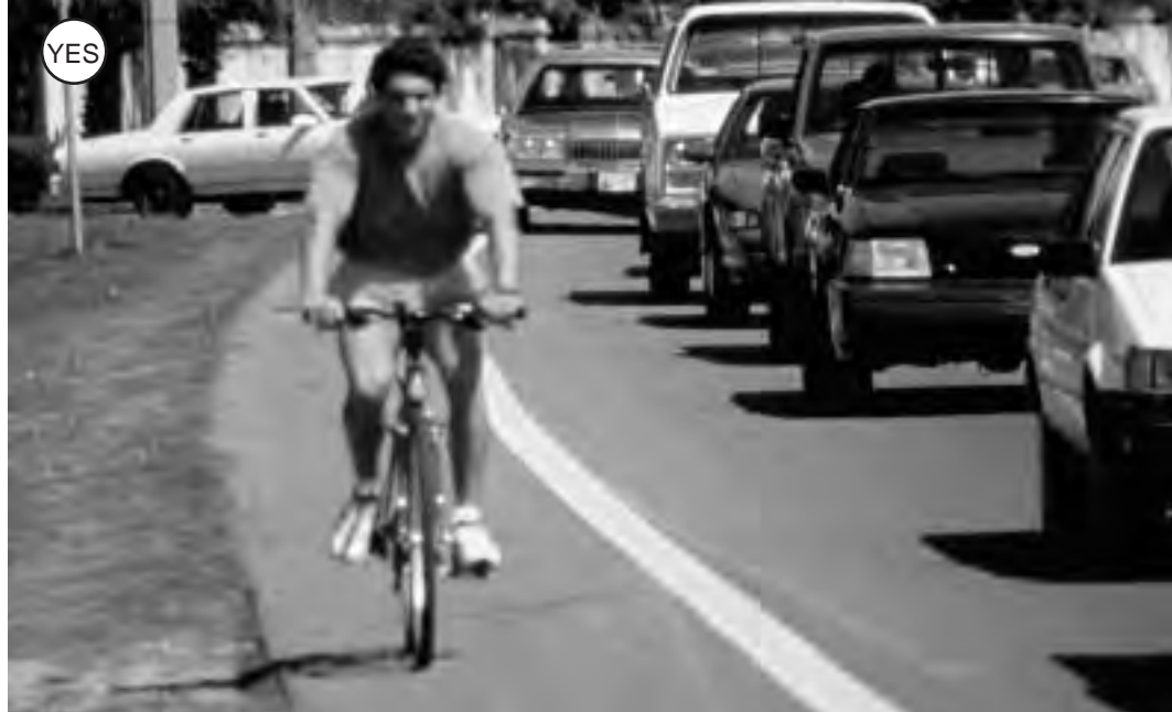
Figure 3-20: Striping bicycle lanes on roadways without curbs can be an important improvement in fast growing suburban and exurban areas.
