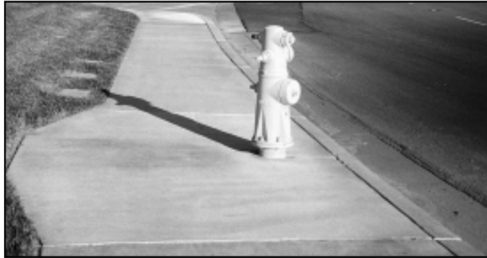
Appropriate sidewalk treatments can accommodate all pedestrians
