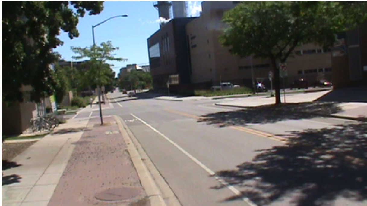
W. Dayton Street looking east toward the study intersection. Image taken from video camera.
