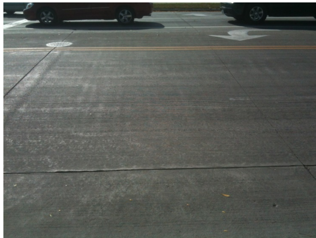
Figure 13. Pictures of typical repaired segments – Project 5 (1420-11-70)
