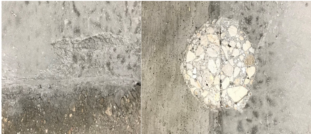
Figure 7.44 – Joint surface prior to (left) and after (right) grinding
