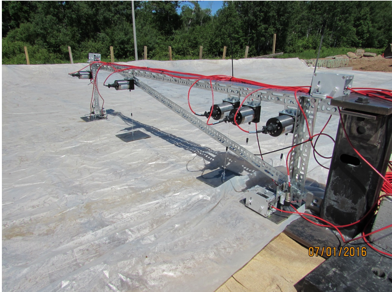
Figure 5.2- Field monitoring instrumentation setup after casting of Stage 2 deck (B-16-136)
