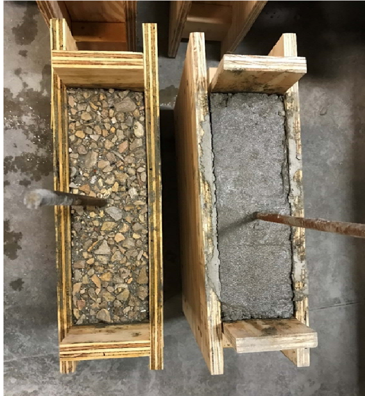
Figure 7.42 – Treated (left) versus untreated (right) joint surface
