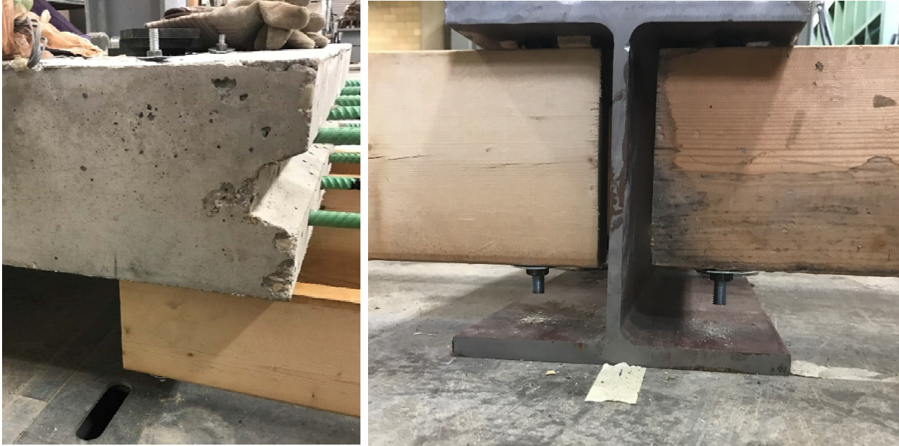
Figure 7.12 - Formwork supporting system connections. Left: steel rod passing through hardened slab. Right: steel rod threaded into nut welded to steel supporting beam.
