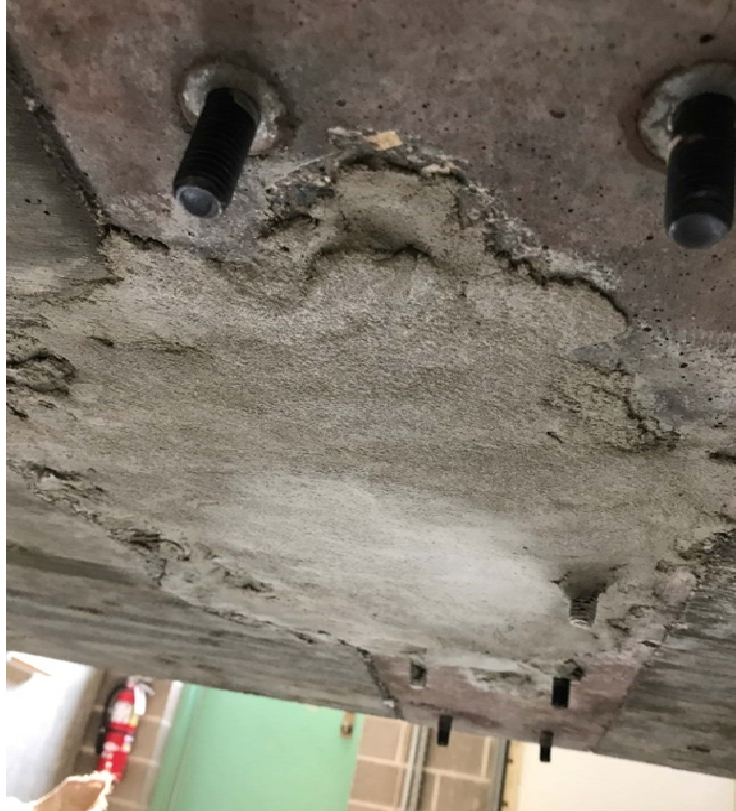
Figure 7.28 - High strength grout repair patch where a shear connector had accidentally been pulled from the underside of the specimen.
