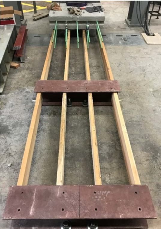
Figure 7.11 - Wood supporting beams in place before plywood is placed on top.
