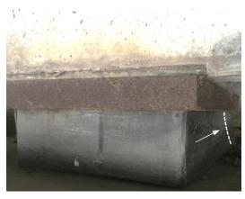
Figure 2.6. Bearing rotation at the obtuse corner. [1]
