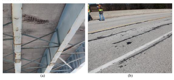
Figure 3.2. (a) Concrete spalling on deck bottom surface for 30° skew, and (b) longitudinal sealed cracks on deck top surface for 3° skew.
