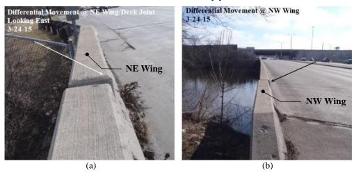
Figure 2.5. Misalignment of wingwall and bridge parapet wall at (a) acute, and (b) obtuse corners. [1]
