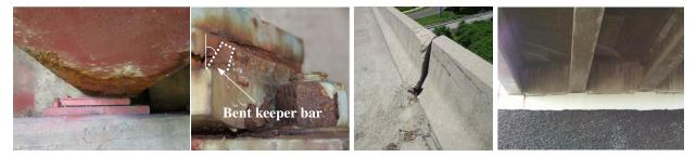
Figure A. Misaligned girder (left), bent keeper bar (middle, left) misaligned parapet wall and closed expansion joint (middle, right), diagonal acute corner deck cracks (right). [1]
