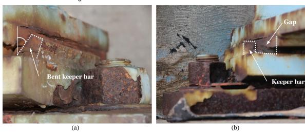
Figure 3.5. (a) Bent interior keeper bar and (b) gap between bearing and exterior keeper bar of obtuse corner bearing at north bridge end for 30° skew.
