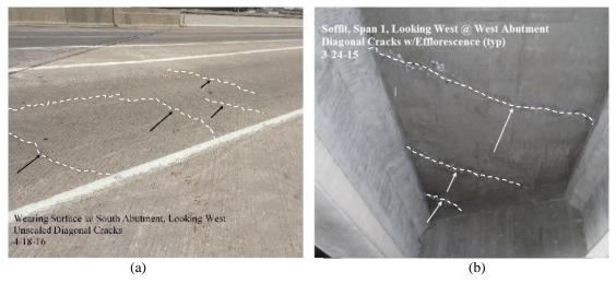
Figure 2.7. Diagonal cracks on the (a) top and (b) bottom faces of the deck at the acute corners. [1]
