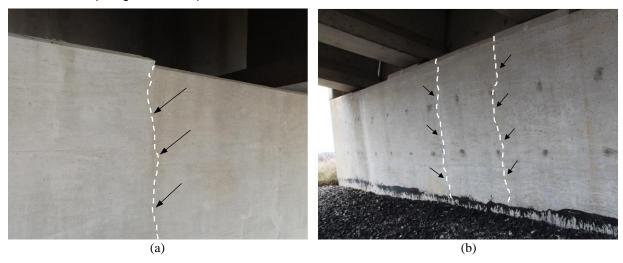
Figure 3.6. Vertical abutment cracks for bridges with (a) 52° skew, and (b) 0° skew.
