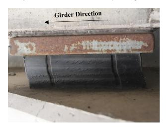
Figure 3.3. Longitudinal displacement of an interior bearing for 52° skew.
