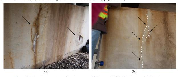
Figure 3.7. Vertical cracks on the abutments of bridges with (a) 30° skew, and (b) 3° skew.
