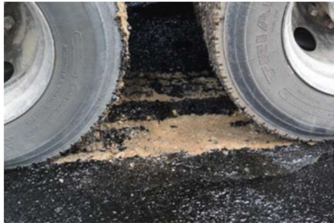
Vehicle tires track tack coat during pavement construction
