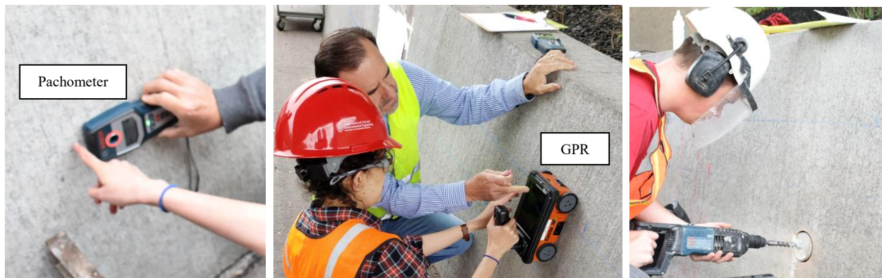
Figure 5.3: Procedure to find the epoxy-coated rebar and connect the electrode to it
