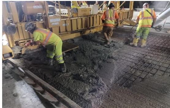
Placement of overlay using double vibrating screed.
