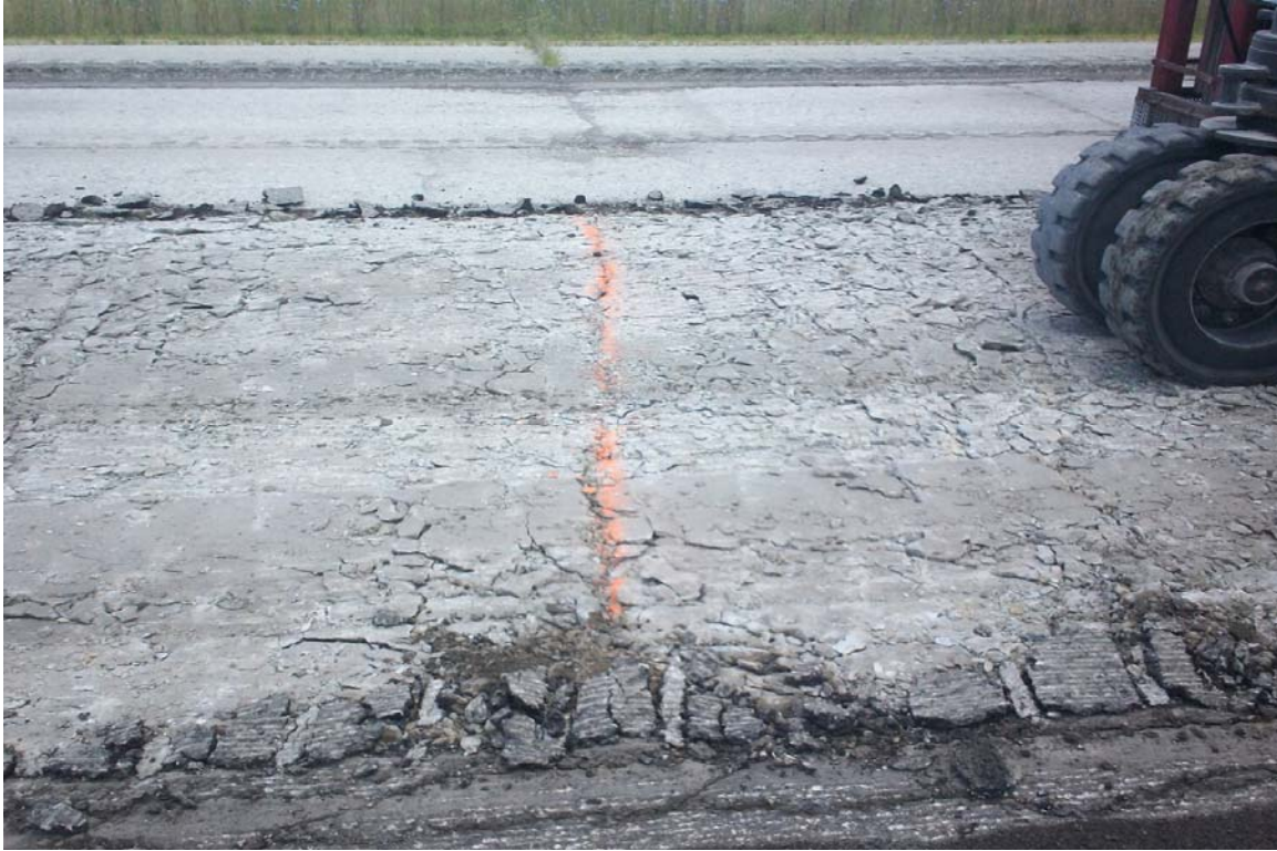
Figure 20. Lower rubblization energy
