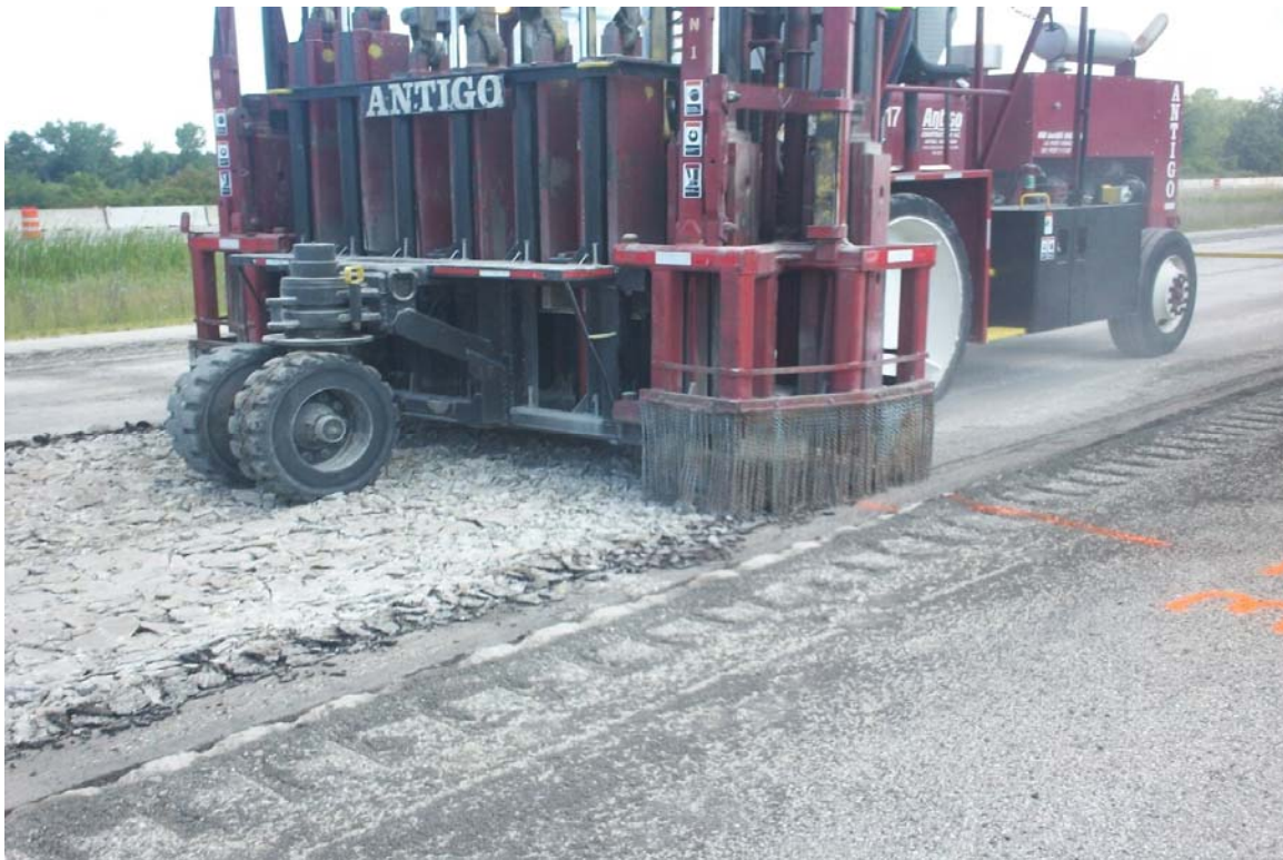
Figure 19. Higher rubblization energy
