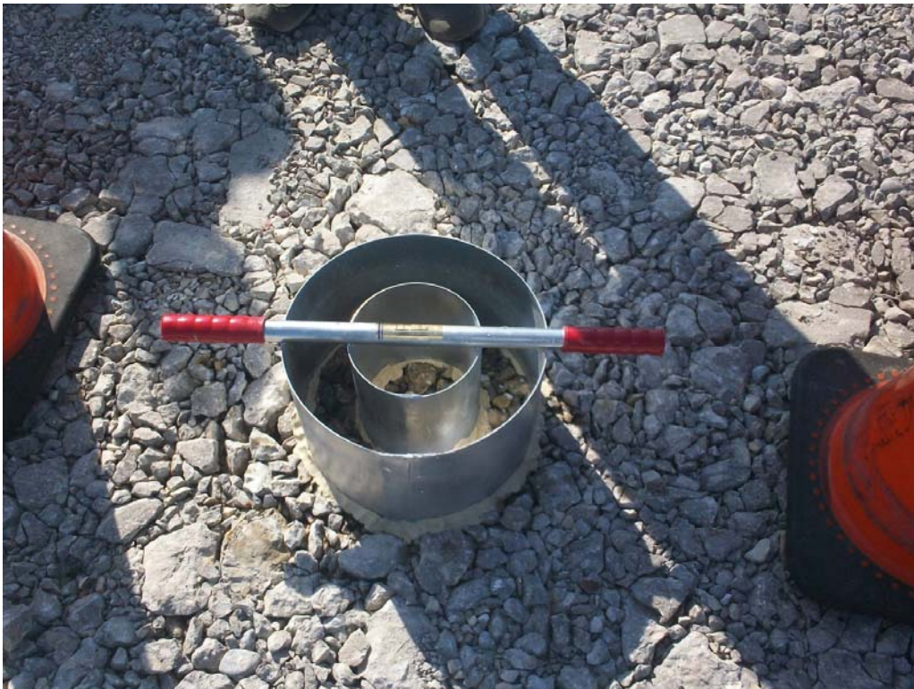
Figure 22. Permeability test setup after test
