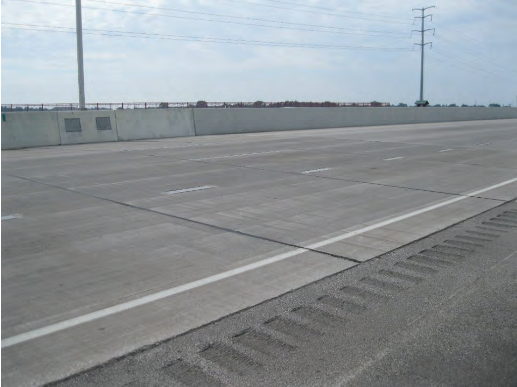
Figure 5-73 B-70-0268 Bridge Approach
