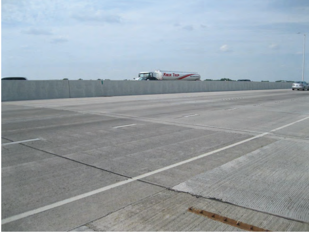
Figure 5-57 B-70-0265 Approach Slab
