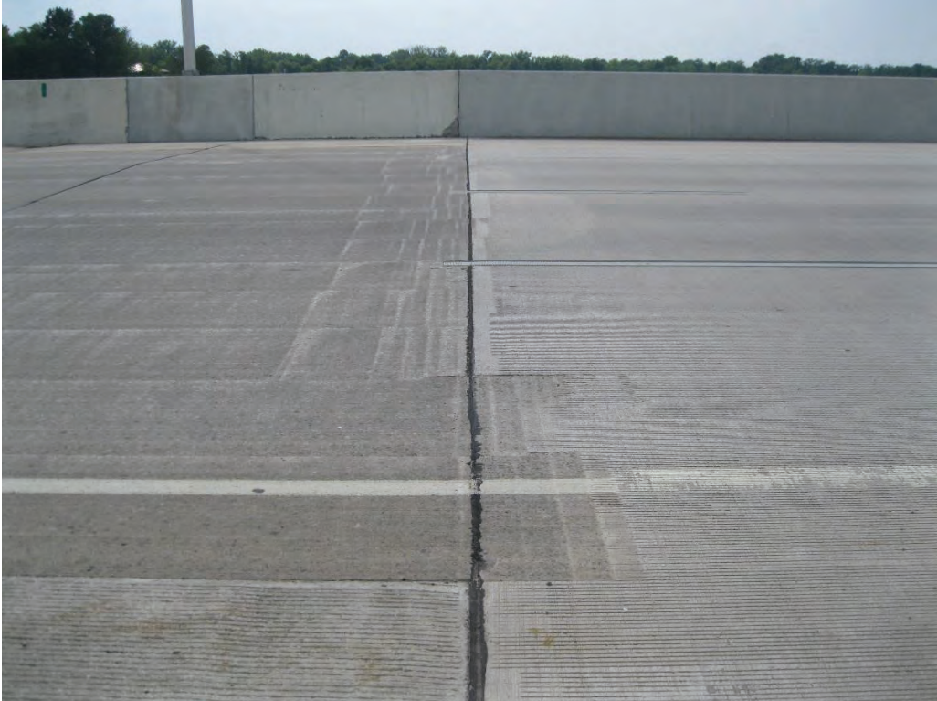
Figure 5-48 B-70-0263 Expansion Joints
