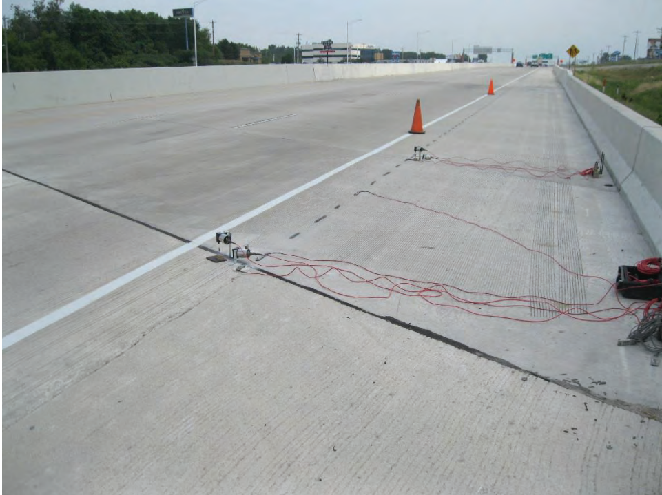
Figure 5-16 B-05-0605 Instrumentation Setup
