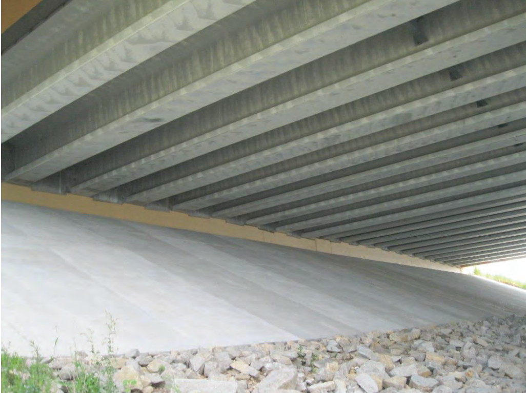
Figure 5-67 B-70-0266 Superstructure Condition
