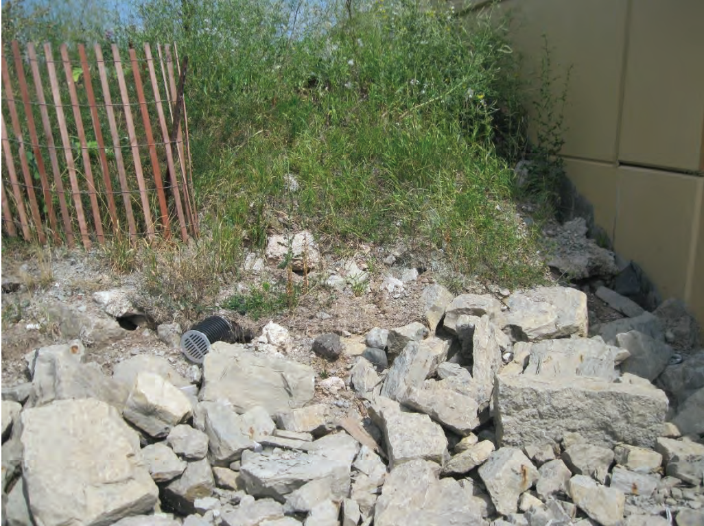
Figure 5-53 Embankment Adjacent to Wingwall
