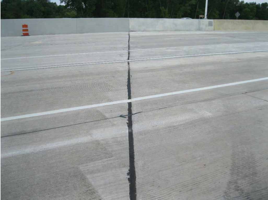
Figure 5-44 B-05-0651 Expansion Joint Condition
