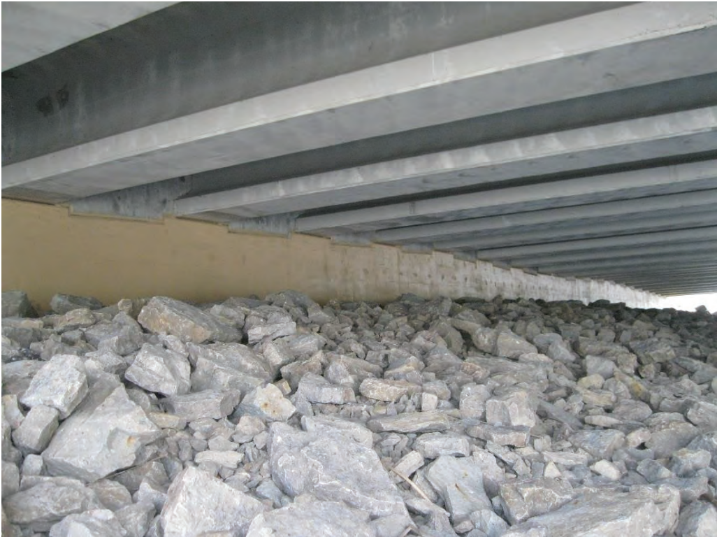
Figure 5-54 B-70-0264 Substructure and Superstructure Review
