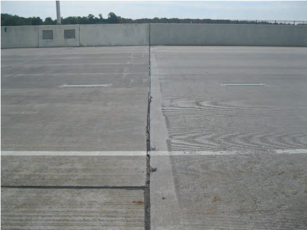
Figure 5-74 B-70-0268 Joint Sealant at Bridge Deck
