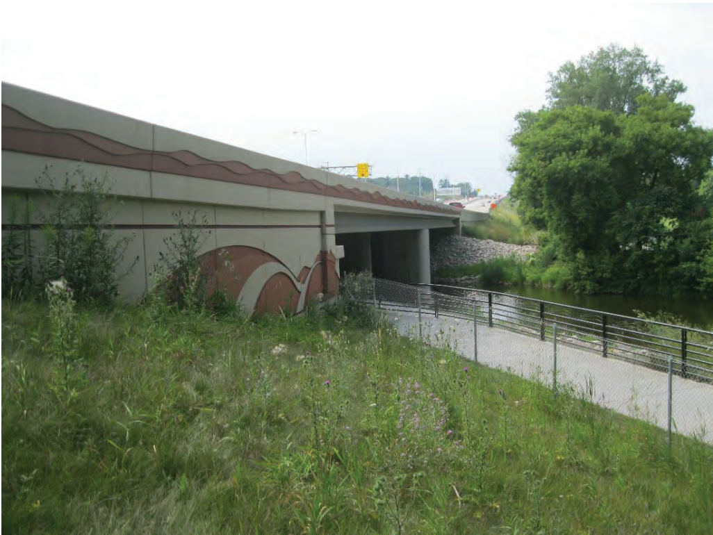
Figure 5-41 B-05-0650 Embankment Slope Adjacent to Wingwall
