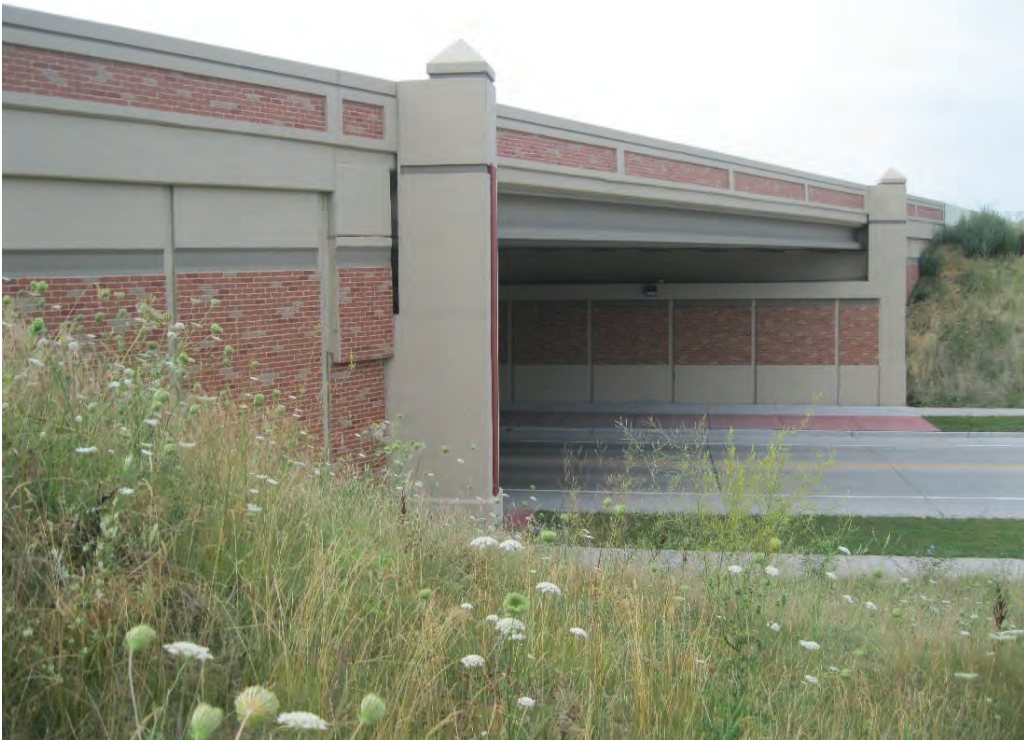
Figure 5-26 B-05-0606 Wingwall Extensions
