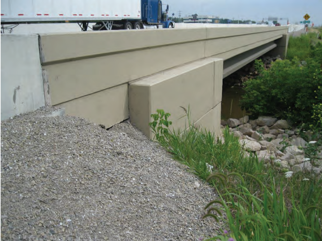
Figure 5-13 B-05-0605 Embankment Condition
