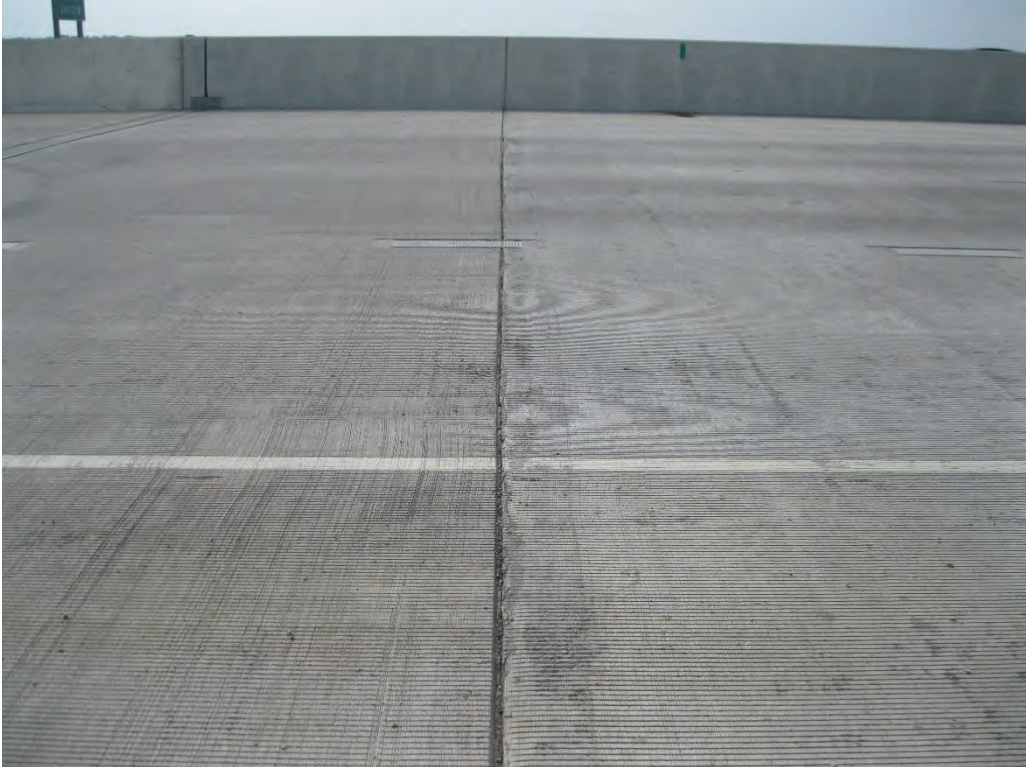
Figure 5-58 B-70-0265 Approach to Deck Joint
