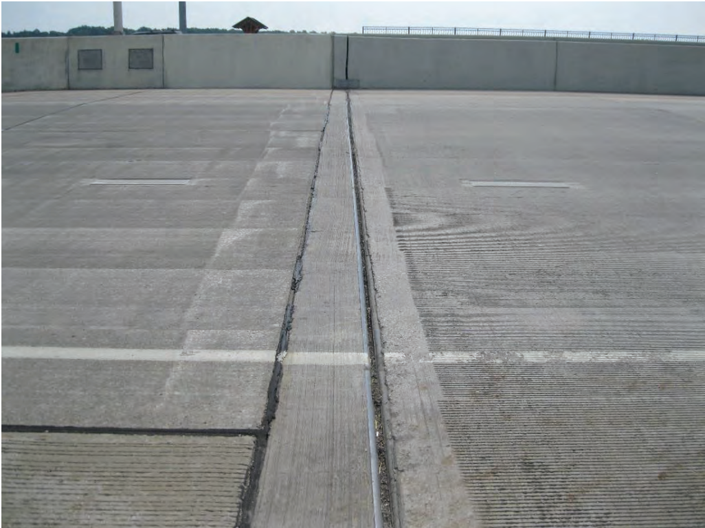
Figure 5-66 B-70-0266 Approach Expansion Joint
