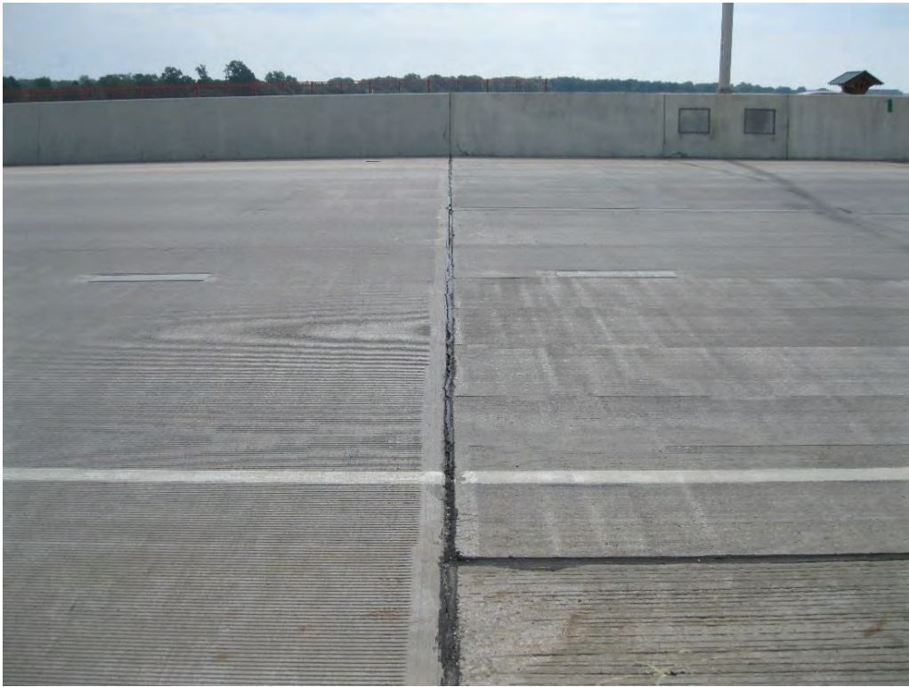
Figure 5-64 B-70-0266 Expansion Joint Condition
