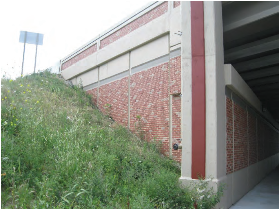
Figure 5-34 B-05-0607 Wingwall extension and embankment condition
