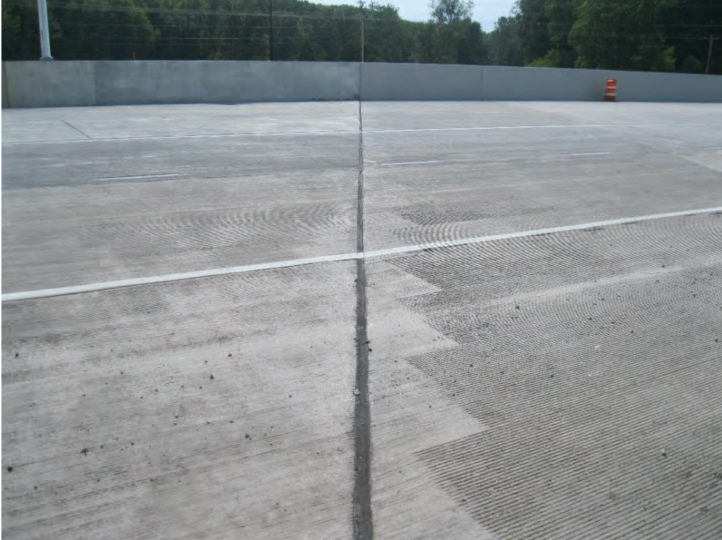
Figure 5-38 B-05-0650 Expansion Joint Condition
