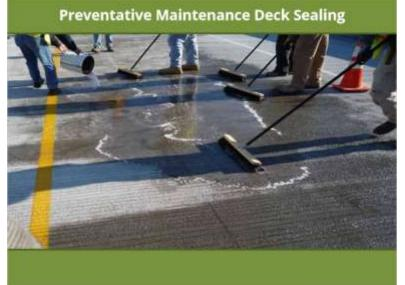
In addition to crack sealing, an important activity to maintain a bridge structure involves deck sealing. Deck sealing involves flooding the deck with an approved sealing product that works to significantly slow the ingress of chloride ions into bridge-deck concrete, thus slowing deterioration of the structure.
