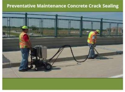
Another common preventative maintenance is crack sealing, particularly in concrete decks.
