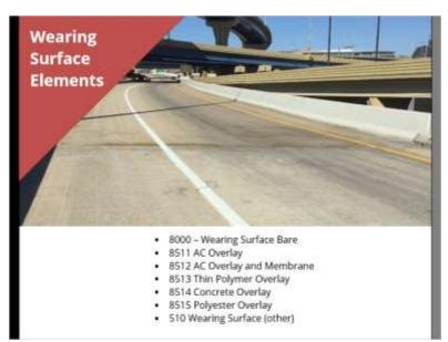
Recall that the top surface of all concrete decks and slabs are evaluated using an associated wearing surface element. If no overlay exists then element 8000, wearing surface –bare is used. If an overlay is present, then the type of overlay (asphalt, thin polymer, concrete or polyester) is coded for the wearing surface.
