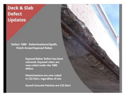
The final change involves patched areas of concrete that are sound. To keep consistent with the AASHTO Manual for Bridge Element Inspections, all sound patches will be coded in condition state 2, fair condition.
