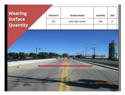
The quantity for the wearing surface would only consist of the portion of the deck that is exposed and not covered by the cantilever sidewalks.ßor this example, the quantity would be the width of 36 feet times the length of 100 feet resulting in 3600 square feet of wearing surface.
