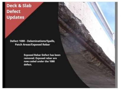
A structure's concrete deck or slab and corresponding wearing surface see more wear and tear than any other component of a bridge due to vehicles and winter de-icing chemicals.
