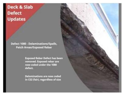
Another change was the language for delaminations. In the 2019 version of the field manual, delamination's are coded in condition state two, regardless of the size of the delamination. This change was made to better mirror the defect language in the AASHTO Manual for Bridge Element Inspections.
