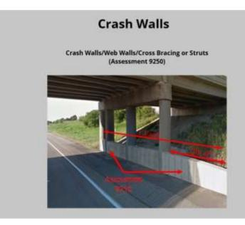
All web walls and most crash walls attached to a pier shall be assessed 20' from exterior columns and coded under (Assessment 9250) The quantity is 1 each per substructure unit.
