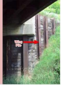
When a bridge has piles supporting the wingwalls, evaluate these piles under the Integral Wingwall Element (8400). Only piles that support the superstructure are to be coded under element 225 Steel Pile.
