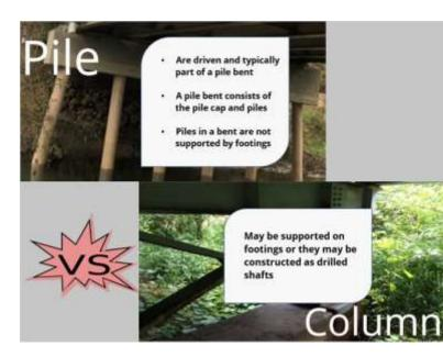
Structural piles are an example of an element commonly miscoded during bridge inspections throughout Wisconsin. Although structural piles function similarly to columns, they need to be coded separately in the element inspection.
