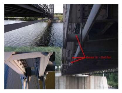
One other connection type consists of steel pins connecting eyebar members. For these situations, the gusset plate element is generally not valid. The inspector should code these using Element 161 for Steel Pins.
