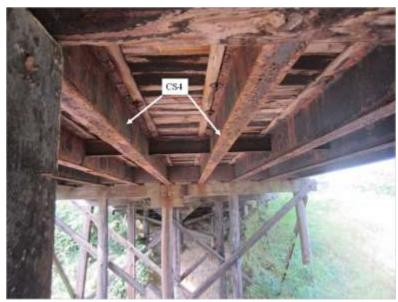
*This example shows a failed paint system, or condition state 4.*
