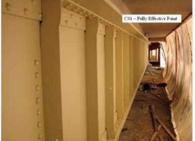
Paint that is in good condition is depicted in this photo. Note that the paint shows no signs of fading nor peeling, and both the finish and primer coats are in excellent condition.
