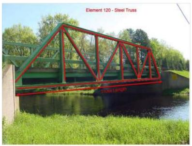
Element 120 encompasses all tension and compression members in the plane of the truss as well as secondary gusset plates in the plane of the truss, and the condition is recorded in units of lineal feet.
