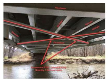
Below the truss deck, the primary superstructure components include: Element 152 Steel floor beams and Element 113 – Steel Stringers which are both recorded in lineal feet.
