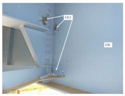
In this example, the paint system is generally in good condition, but has spots where the finish coat is starting to peel away from the still fully-intact primer coat. These isolated areas would be coded in fair condition (CS2) while most of the paint system would still be in Good condition (or CS1).
