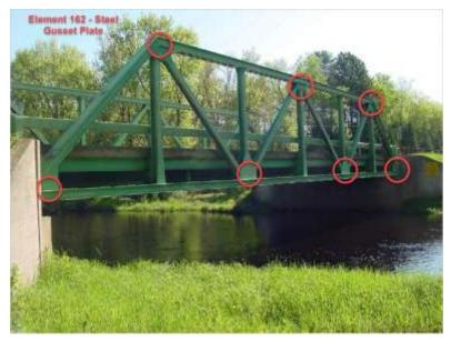
Gusset plates are typically used to connect truss members together, most commonly with bolts or rivets. They are constructed of one or more steel plates and are documented in Each units on the inspection form.
