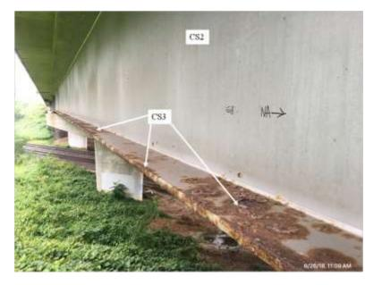
A common location for paint deterioration is on the bottom flange. This is due to several factors including the flat flange surface capturing salts, moisture and debris. In addition, on sharp corners such as the edge of flanges, there is potential for the paint to be thinner due to difficulties in application.
