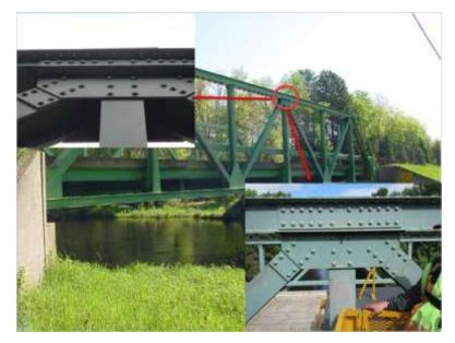
Typically a panel point connection consists of two plates, one on the roadside of the truss and one on the exterior of the truss. This assembly is counted as a quantity of one on the inspection report.
