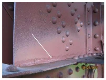
Another important tip to remember is that an element with measurable section loss where the defect is in condition state 3 or 4 for corrosion will still be in that same condition state after it has been repainted. Only the paint effectiveness element will be reverted back to a good condition state. The paint only covers up the section loss; it does not fix it.
