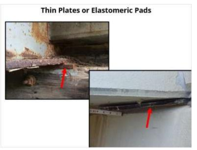
There are several types of movable steel bearings that are used to support bridge superstructures. These include rollers, rockers, and sliding plates. Movable bearings are designed to accommodate superstructure expansion, contraction, and rotation.
