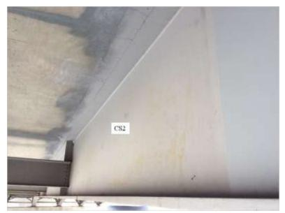
This is another example of the fair condition state (or CS2). As can be seen in the photo, most of the web of this girder has blush rust (or sometimes called freckle rust), but for the most part the paint system is performing its intended function.
