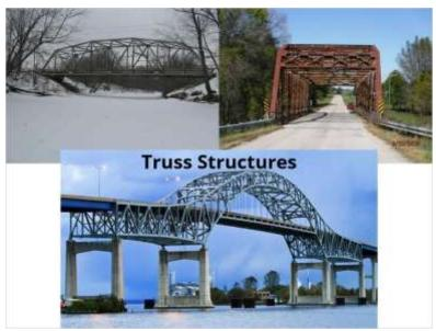
Steel truss bridges were commonly built in the early to mid 1900's due to the ability for these structures to span long distances. As advances in technology allowed for steel girders and later prestressed girders allowed for longer and longer spans, the truss structure became mostly obsolete.
