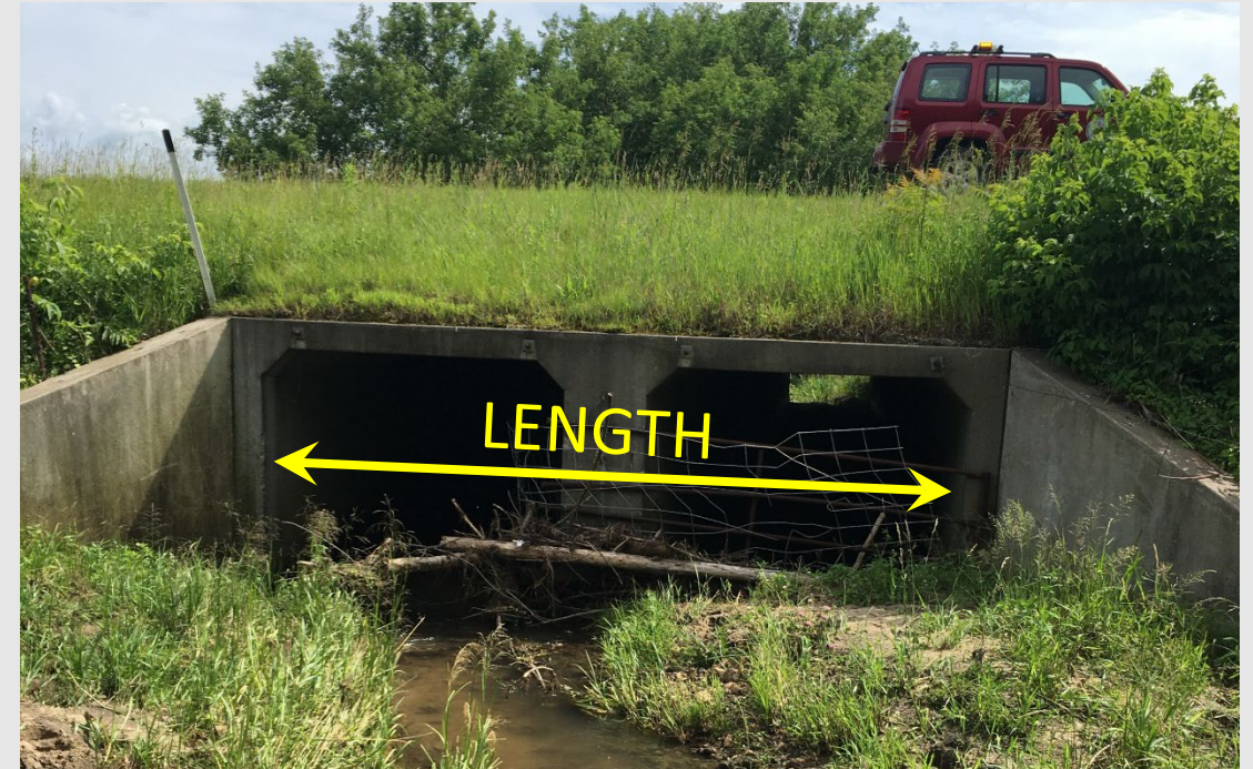
Double Barrel (multicell) Box Culvert
