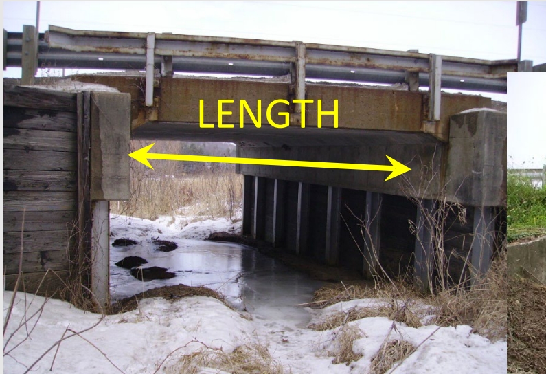
Concrete Flat Slab
