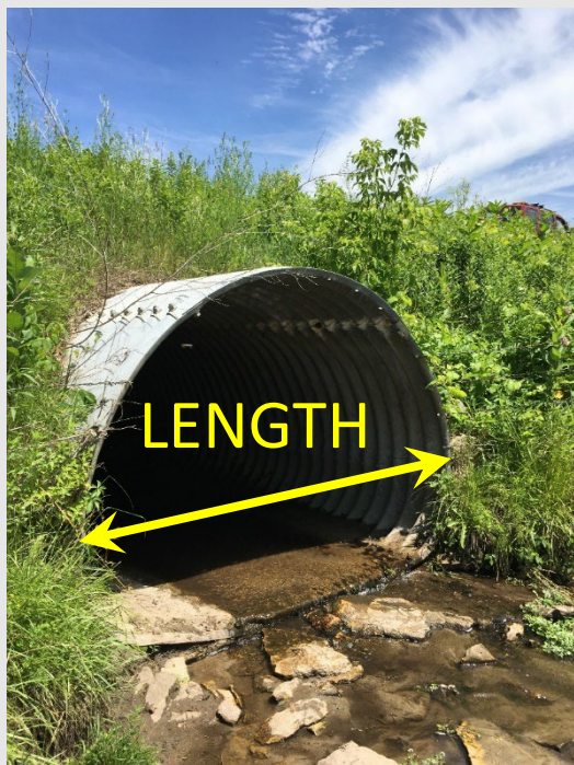
Steel Pipe Arch
