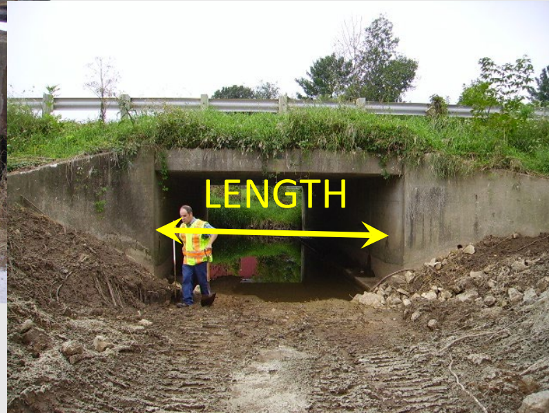
Buried Rigid Frame (no floor)
