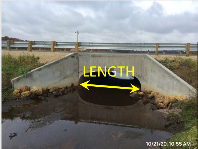
Precast Concrete Arch
