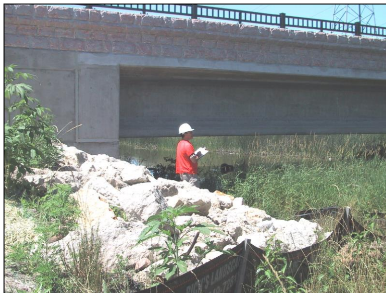
Figure 1.3.2.1-1: Inspector Performing an Initial Inspection.
