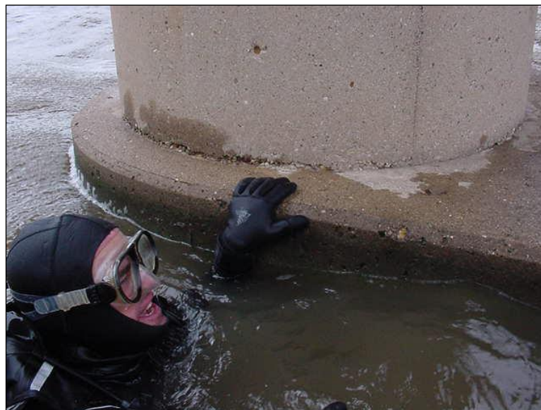
Figure 1.3.8.2-2: Inspector Conducting a Level I Inspection Effort.
