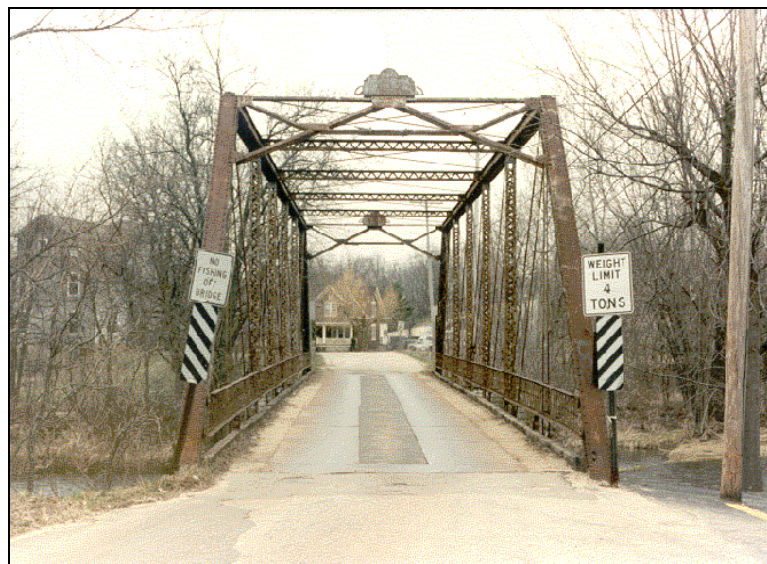
Figure 1.3.13.1-2: Load Posted Truss Bridge.
