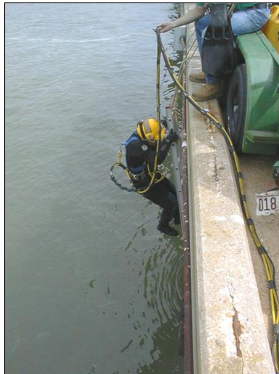
Figure 1.3.8.4-1: Inspector Using Surface-Supplied Air Equipment.
