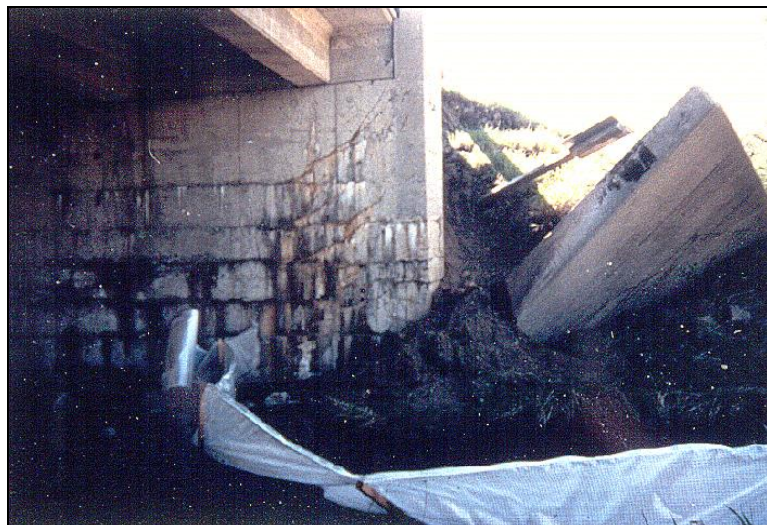
Figure 1.3.12.1-2: Failed Wingwall.
