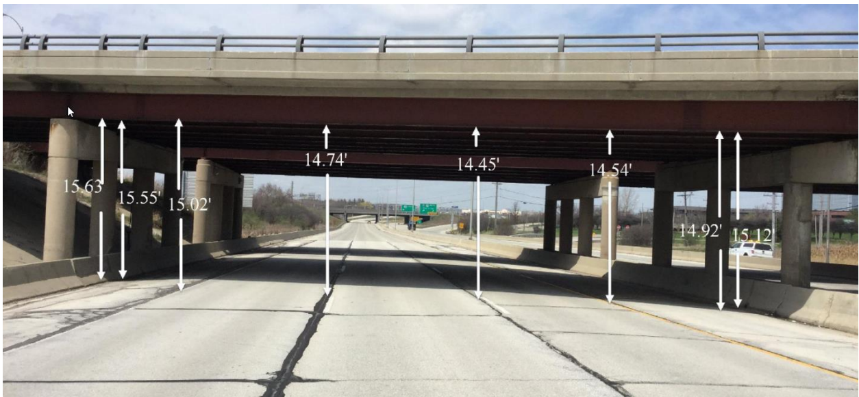
Figure 1.3.15.1-1: Vertical Clearance Photo
