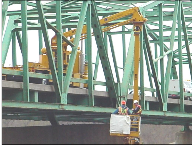
Figure 1.3.5.1-1: Inspectors Performing an NSTM Inspection
