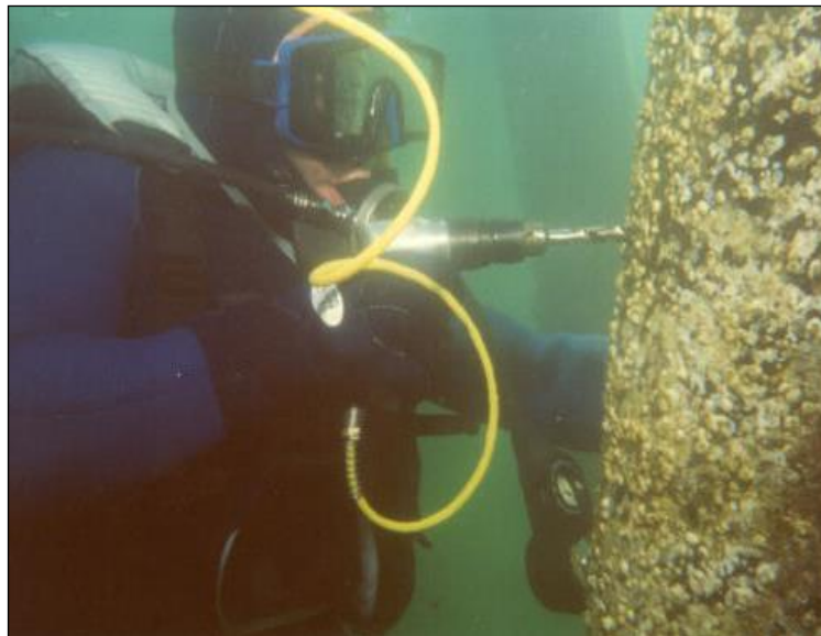
Figure 1.3.8.2-5: Inspector Using a Drill to Conduct a Level III PDE Inspection Effort.
